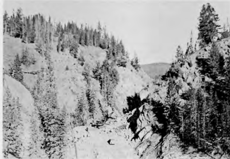
Construction of Flint Cr. Hill road
