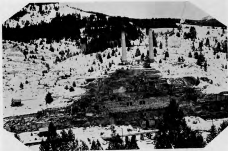
Bi-Metallic Mill after controlled burn
