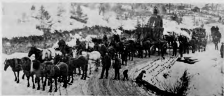
Transporting motor casting to Granite City, 1902
