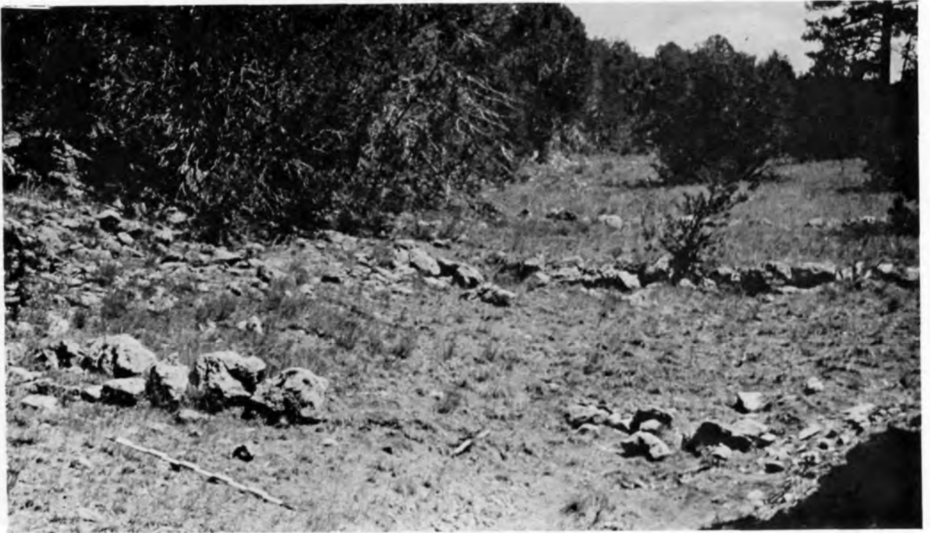
Figure 34. Check dams in the Chevelon area.
