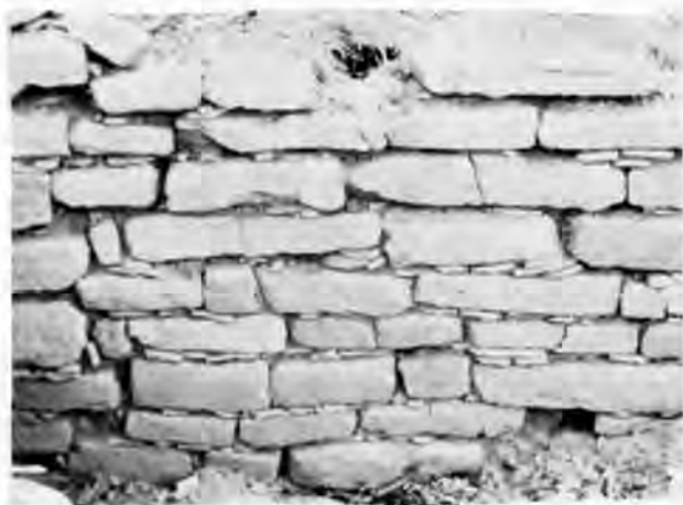
Figure 53. In the Pinedale area, walls exposed in potholes are often the only evidence of Pueblo architecture.
