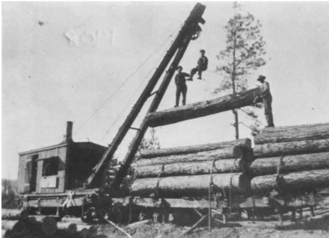
Figure 55. Loading stopped for the photographer in this image, taken circa 1908 near Sawyer. The obvious casual attitude with regard to the heavy load and the lack of safety equipment would not be allowed by modern safety engineers. ( John Bigley collection )
