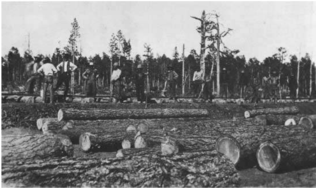
Figure 65. Zuni Mountain Railway track gang comprised mostly of Navajo Indians. The track is not yet ballasted, and is laid on a newly graded roadbed. ( Cibola National Forest collection )
