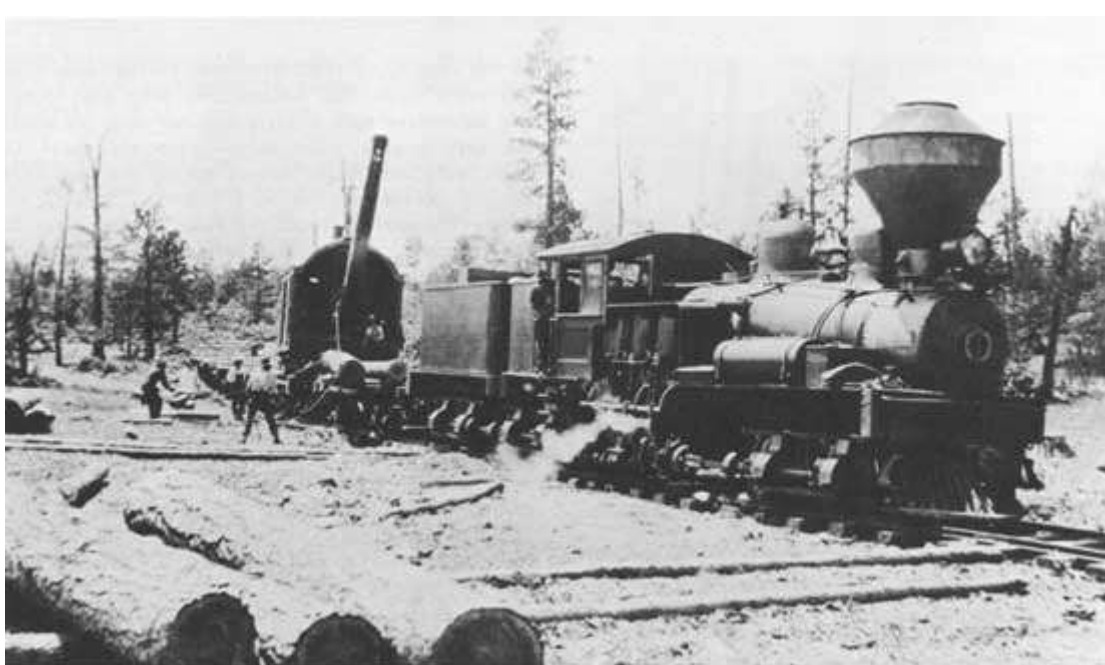
Figure 39. Loading logs on the McGaffey Contracting Company cutting. Shay locomotive Number 1 waited while the Barnhart loader hoisted the 16 to 20 foot pine logs onto the cars. After each car was loaded, the loader moved back one car length to repeat the process. The loader rode on car-top rails.
