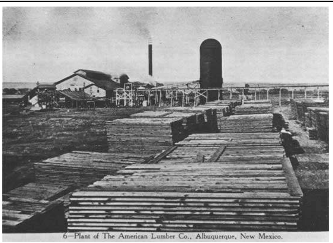
Figure 4. Sawmill, sawdust burner, and lumber storage yard of the American Lumber Company at Albuquerque, New Mexico, in the early years, circa 1903-1904. ( V. J. Glover collection )
