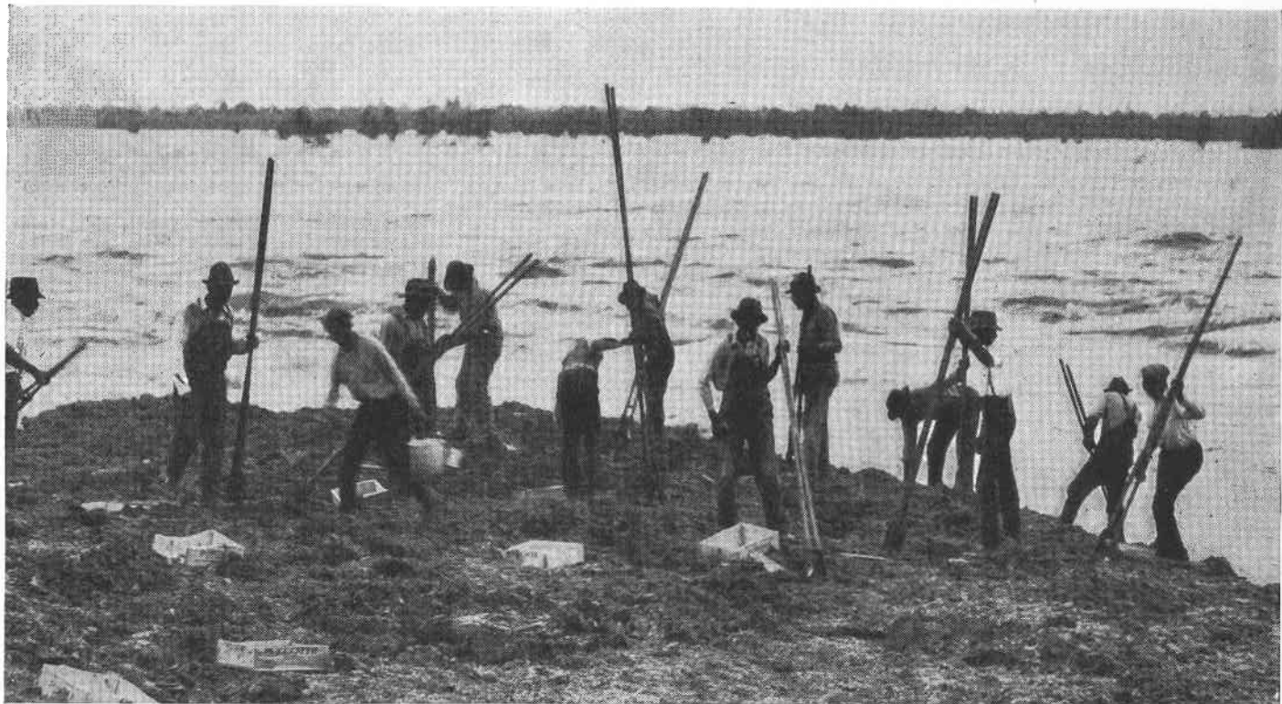
Working on the Mississippi Levee
