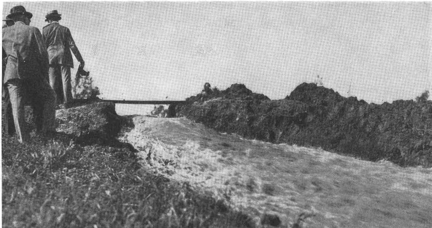
The Levee Breaks!
