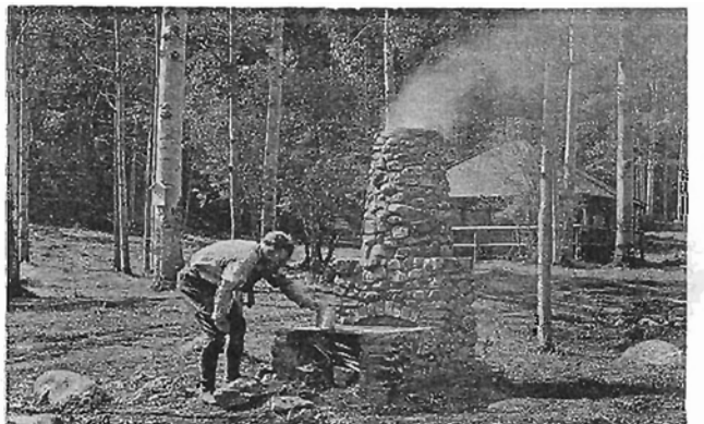
Figure 11.—Stone masonry fireplace with fixed metal cooking lid. Picnic shelter with central fireplace in background. Ophir Creek campground, San Isabel National Forest, near Wetmore, Colo., 1925.
