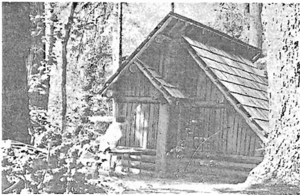
Figure 24.—This 1936 camper's shelter is larger than the simple Adirondack-style shelters shown in figure 8, and has counter, bench, and enclosed cupboards not found in those shelters. McKenzie Bridge camp, Willamette National Forest, Oregon.
