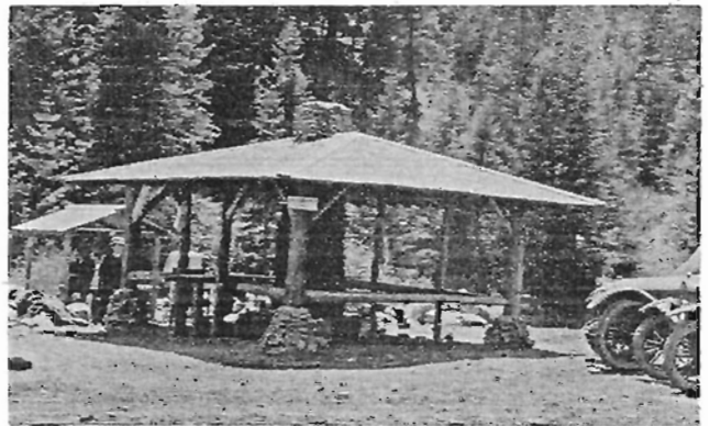
Figure 9.—Simple picnic ground shelter with central stone masonry fireplace, built with funds raised by residents of Pueblo, Colo., on Squirrel Creek, San Isabel National Forest, in 1918, for use of general public.
