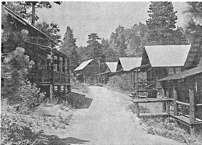
Figure 4.—Summer cabin community in San Bernardino Mountains in 1916, under lease on National Forest land. This section became part of the San Bernardino National Forest in 1925. Term Lease Law of 1915 greatly stimulated summer and resort building on Federal lands.
