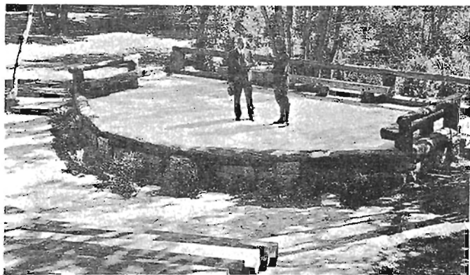
Figure 19.—Concrete stage and split log seats of amphitheater built by CCC in Box Elder Picnic Area, Wasatch National Forest, Utah, 1936. High stone masonry wall was added to back of some such structures at this time.
