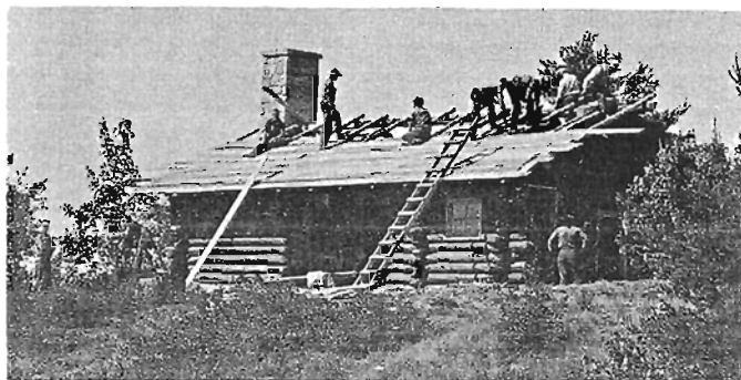
Figure 18.—Log bathhouse under construction with Civilian Conservation Corps labor in 1936 at Soldier Lake, Marquette National Forest, Upper Michigan (since 1962 part of Hiawatha National Forest). Many sizes and styles in cedar shingle, clapboard, and stone were built on National Forests during this period.
