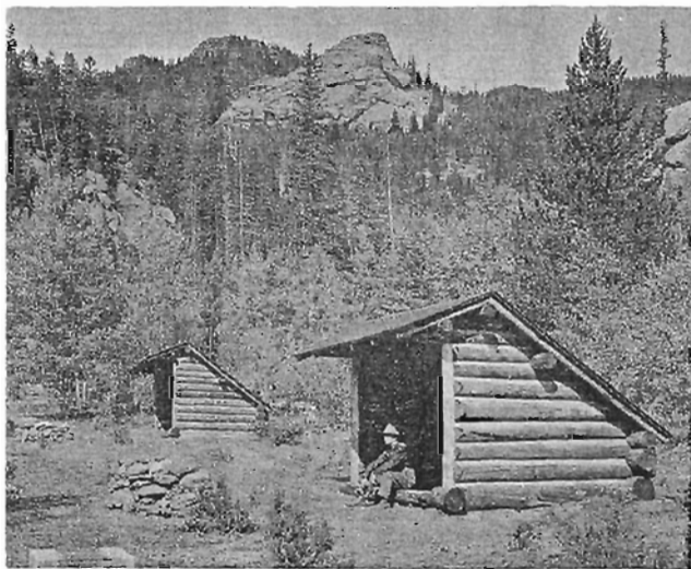
Figure 8.—These Adirondack-style log shelters were installed at Beaver Meadow campground, Pike National Forest, Colo., in 1917, and elsewhere later. Simple lean-to trail shelters were in use on National Forests in Oregon and Washington by 1916. Note loose stone warming fireplaces in front, and low metal cooking grills embedded in concrete sides.
