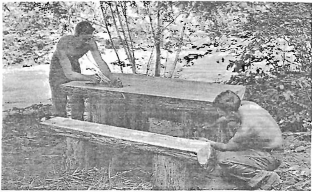
Figure 23.—Picnic table and bench made of split cedar logs by CCC labor, 1936. Eagle Creek campground, Mt. Hood National Forest, Oregon.
