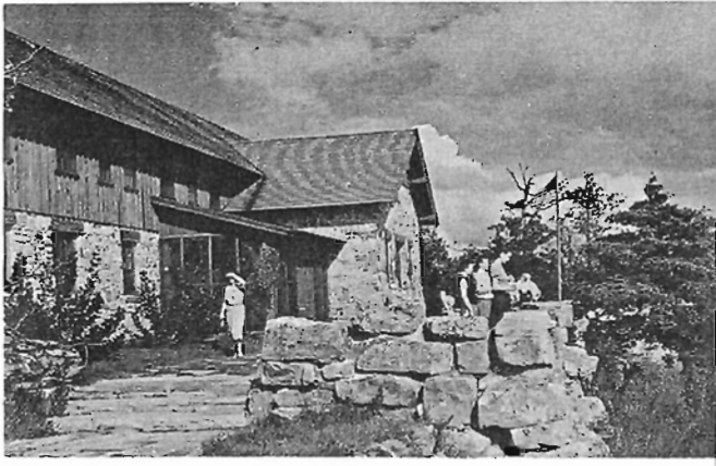
Figure 29.—Mount Magazine Lodge, Ozark National Forest, Ark., was built by WPA in 1939 and operated for the Forest Service under a concession contract for many years. It is the highest point between the southern Appalachians and the Rockies. The Forest Service also operated a number of cottage resorts throughout the South during this period.
