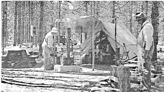
Figure 14.—Camping unit in use, Buffalo Creek site, Targhee National Forest, Idaho, at Island Park Reservoir, major recreation center near Yellowstone National Park. Each unit was provided with picnic table, chopping block and wood, metal stove on concrete platform, and cleared tenting space. Metal stoves were often encased in stone and mortar for natural effect. Note car parked in lot to the rear, preserving ground vegetation. August 1935.
