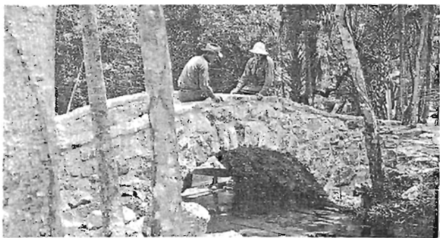
Figure 16.—Stone foot bridge on Ocala National Forest, Florida, 1936.
