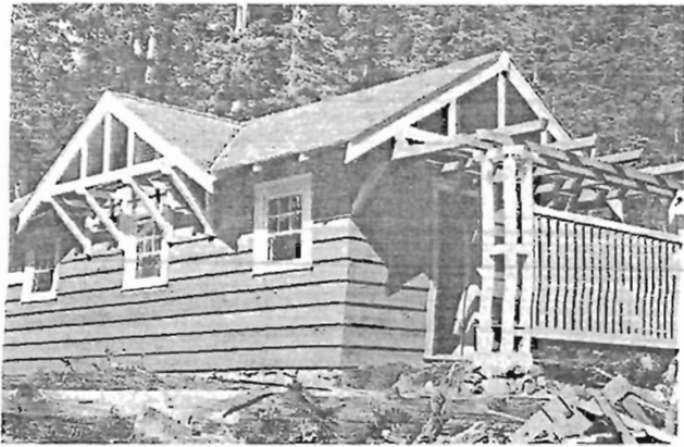
Figure 6.—This restroom was built in 1916 at Eagle Creek campground, Oregon National Forest (renamed Mt. Hood in 1924), along the Columbia Gorge Scenic Highway east of Portland. It is probably the first substantial unit of this kind built by the Forest Service. Many sizes and styles in shingle, clapboard, log, and stone masonry appeared on National Forests throughout the country during the next 25 years. Chemical and flush toilets came late in the 1930's at the most densely used sites.
