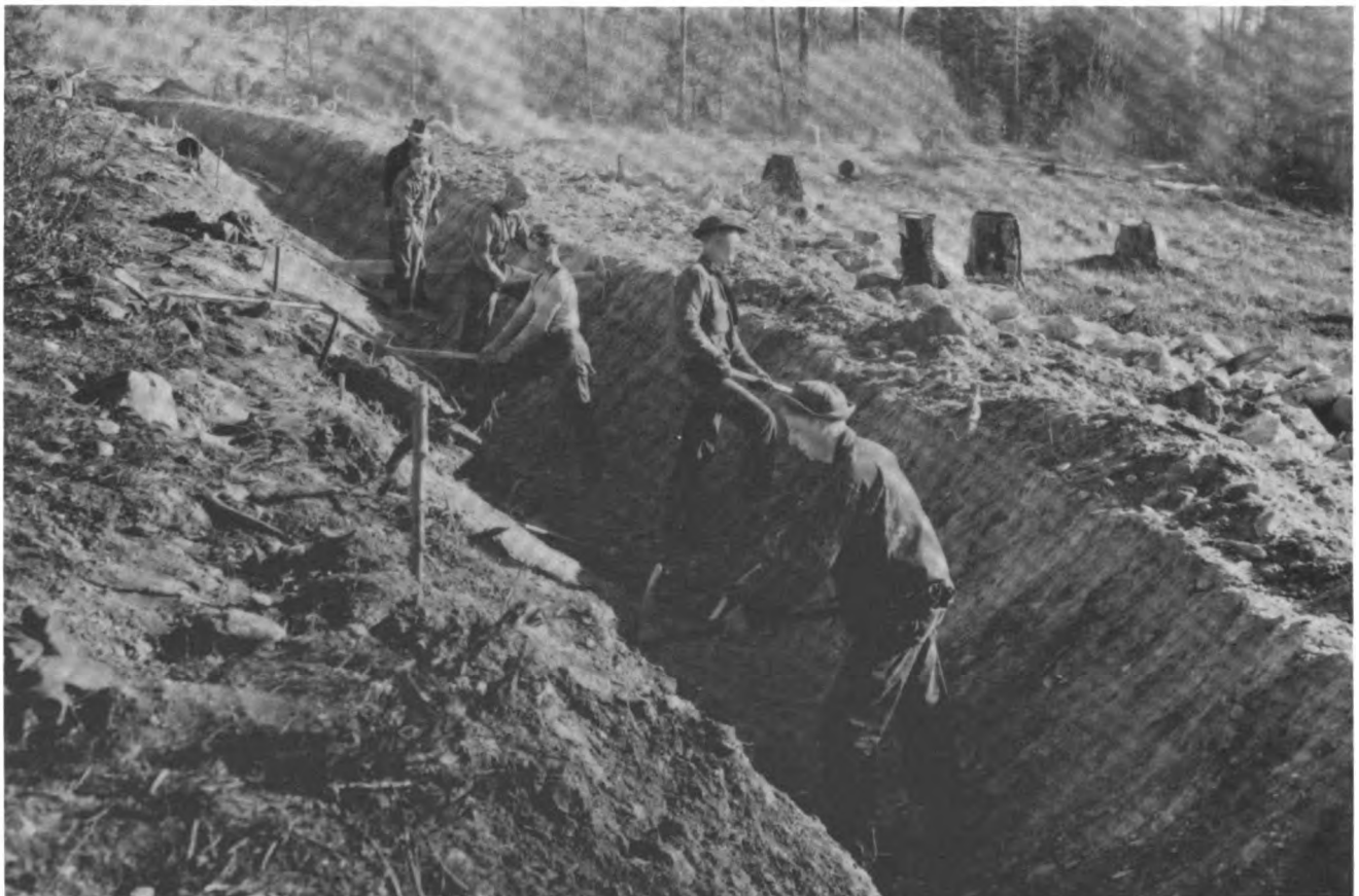
Civilian Conservation Corps Crew digging irrigation ditch for hay lands at Remount Depot, Lolo National Forest, 1934.
