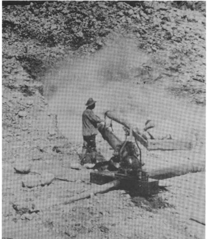
Powerful pump used in hydraulic mining in Idaho during last decades of the 19th century.
