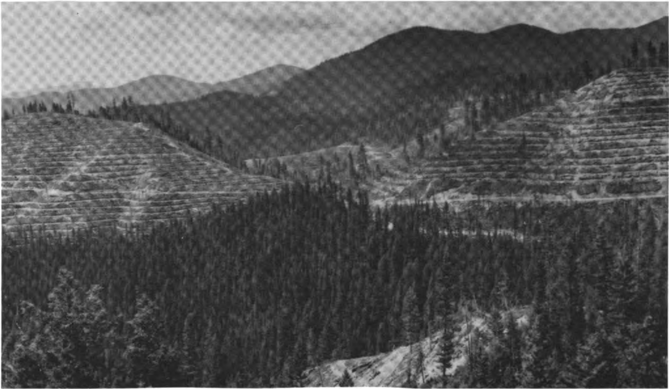
Experimental terraces constructed for tree planting on steep slopes, Bitterroot National Forest.
