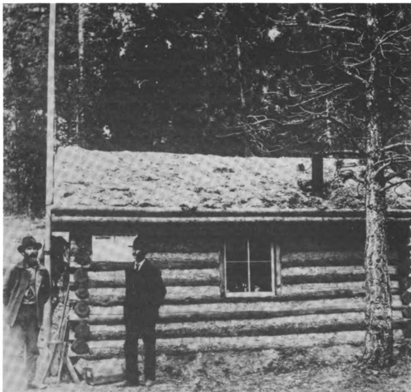
The Alta Ranger Station on the Bitterroot National Forest in Montana, built in 1899, is the first/oldest in the Northern Region. Photo by USDA Photo Service.
