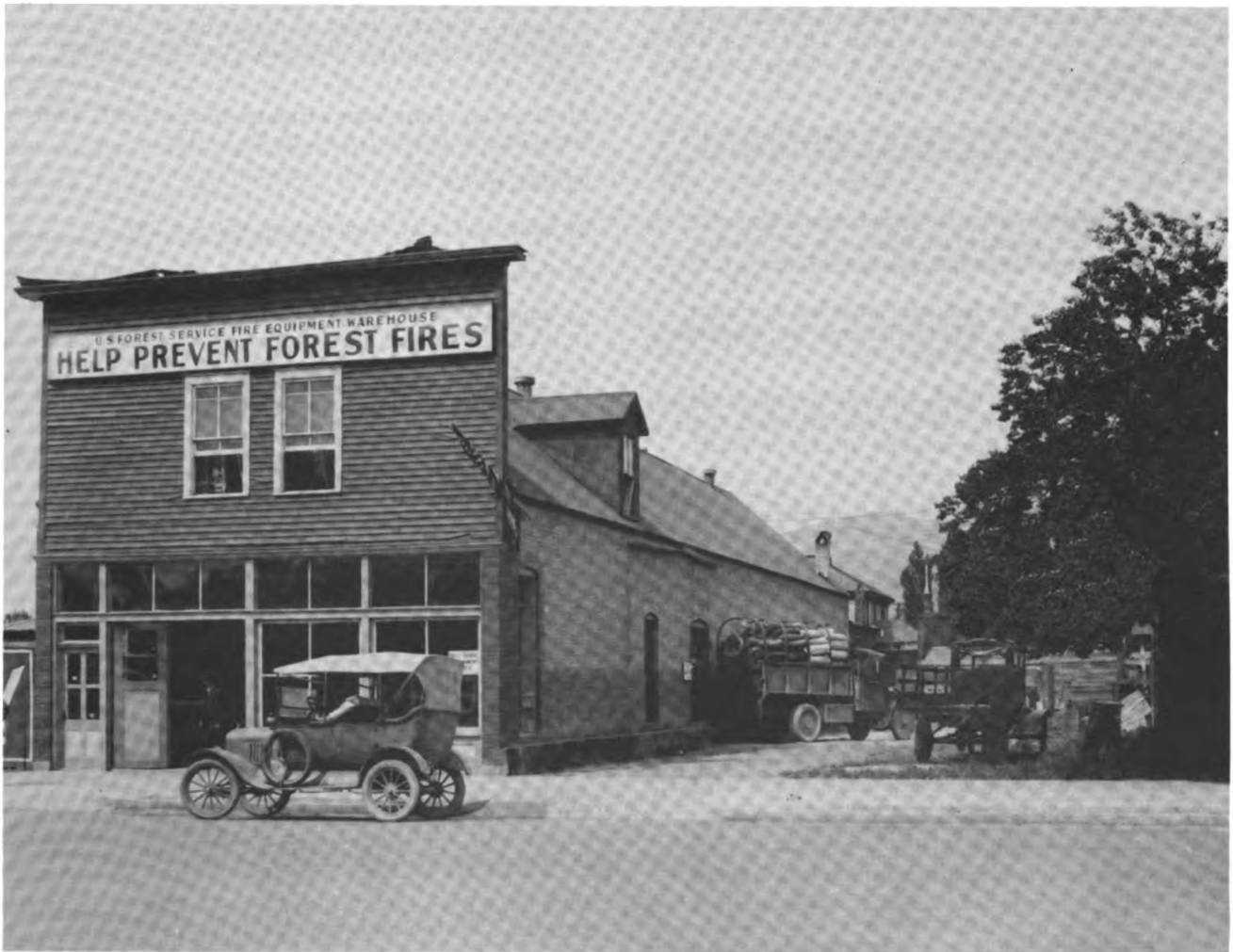
Northern Region Fire Warehouse, Missoula, Montana, 1922.
