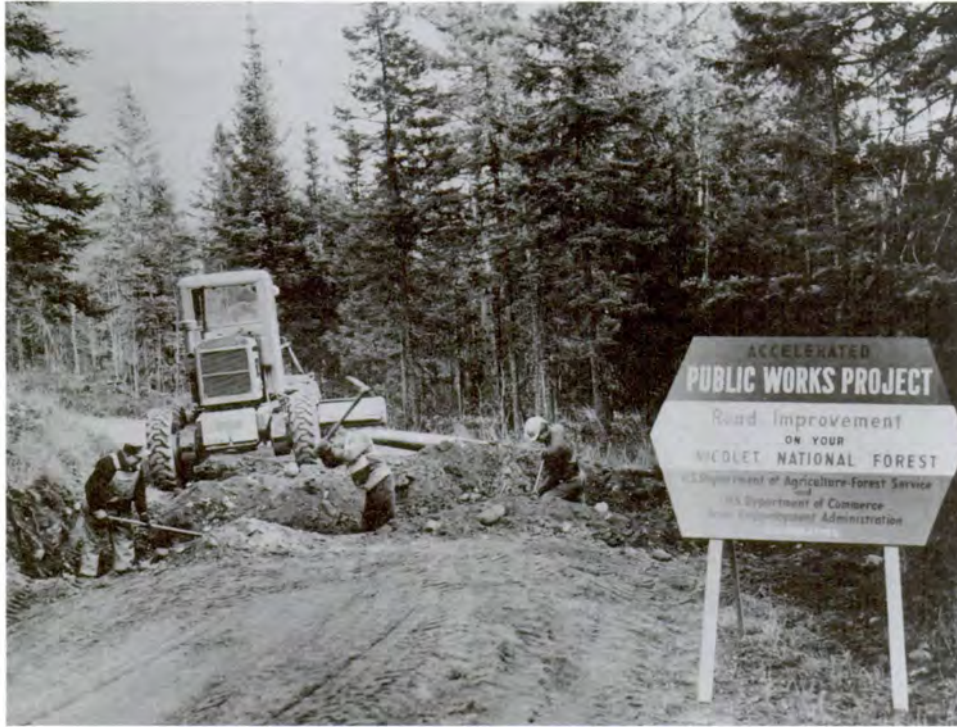
Accelerated Public Works Project workers laying a culvert on Alvin Creek Road, Eagle River Ranger District, Nicolet National Forest, Wisconsin, 1963.
