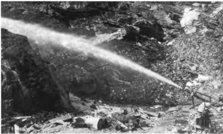
Hydraulic gold mining in operation at Scotts Bar, Klamath National Forest. 1930
