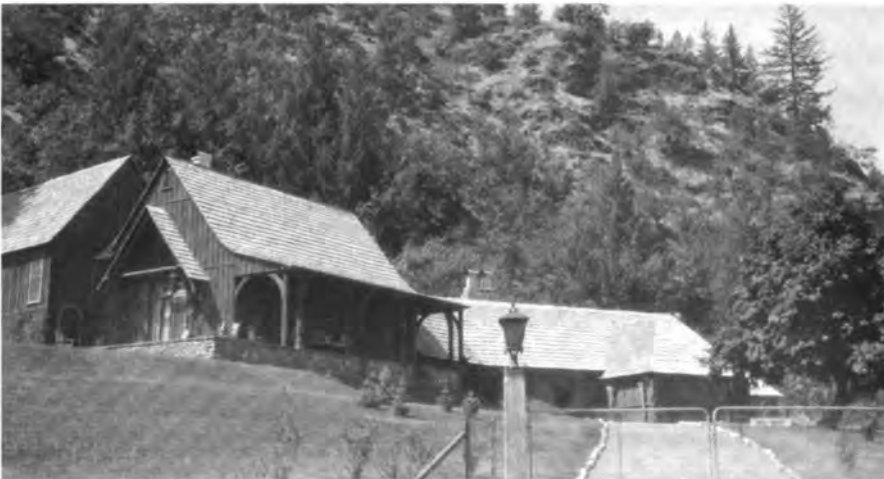
Summer home “improvements” on patented Oak Bar placer claim, Klamath National Forest. 1935
