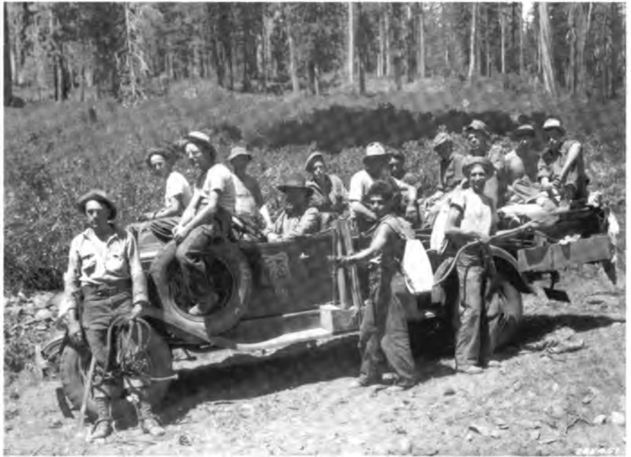
A CCC fire suppression crew on the California National Forest. 1933
