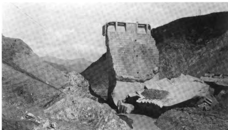
St. Francis Dam after collapse in spring of 1928. Angeles National Forest
