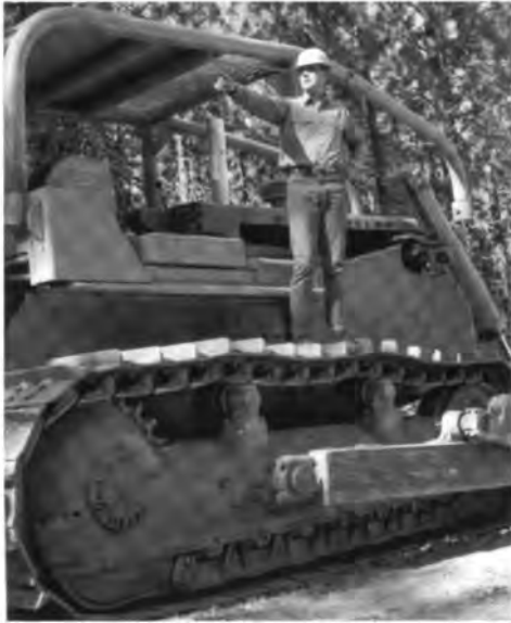
Caterpillar tractor and operator. Soup Creek Timber Sale, Modoc National Forest. 1963
