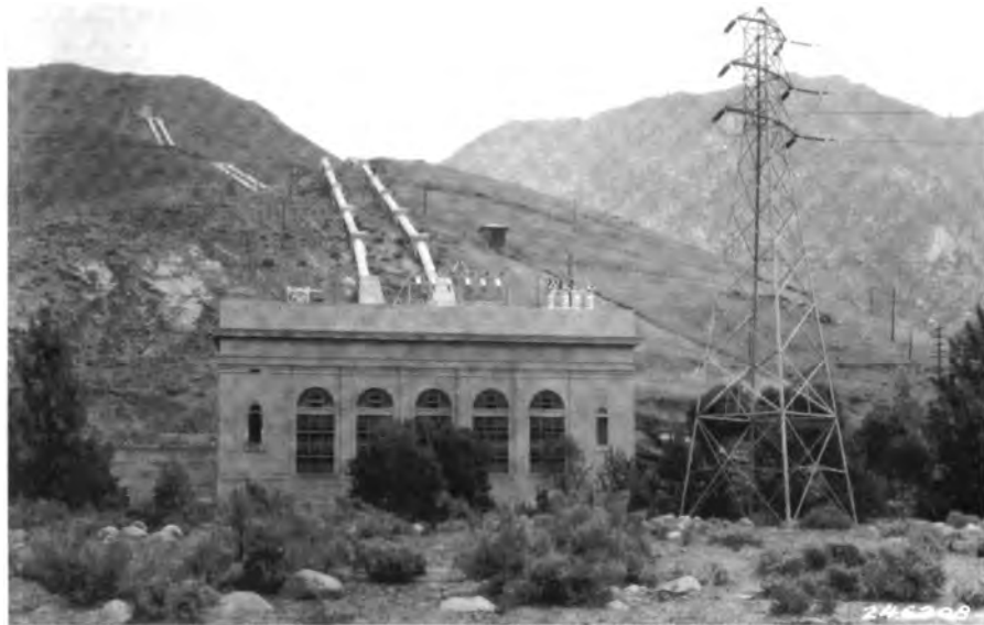
Kern River hydroelectric power plant #3, in Southern California. Sequoia National Forest. 1930
