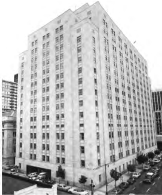
U.S. Appraisers Building on Sansome Street in San Francisco, California. This building was home to the Regional Office until 1998.
