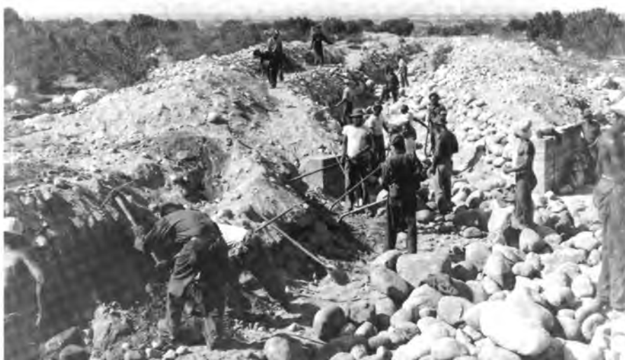
Santa Ana Cone ECW Camp F-153. Enrollees working on water ditch abutments, San Bernardino National Forest. 1933
