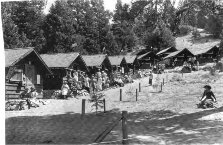
Cottages at the Los Angeles Municipal Camp in the Angeles National Forest. 1926
