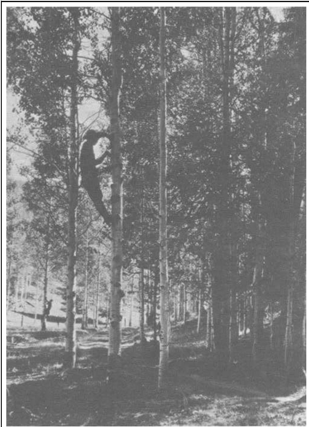
Figure 6. Stringing telephone line on trees on the Kaibab National Forest. Photo by E. S. Shipp dated September 1930.
