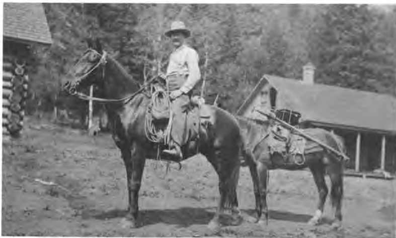
Figure 33. Ranger Stewart, circa 1914, with a mountain telephone packed for transport at Panchuela Ranger Station, Pecos N.F.
