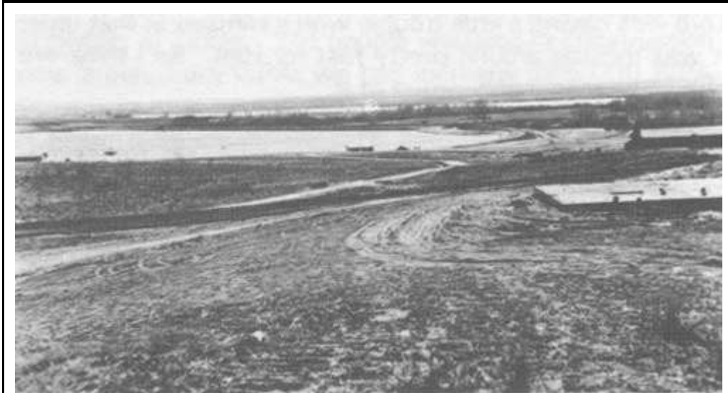
Figure 30. Lake Marvin, shortly after construction, in 1948.
