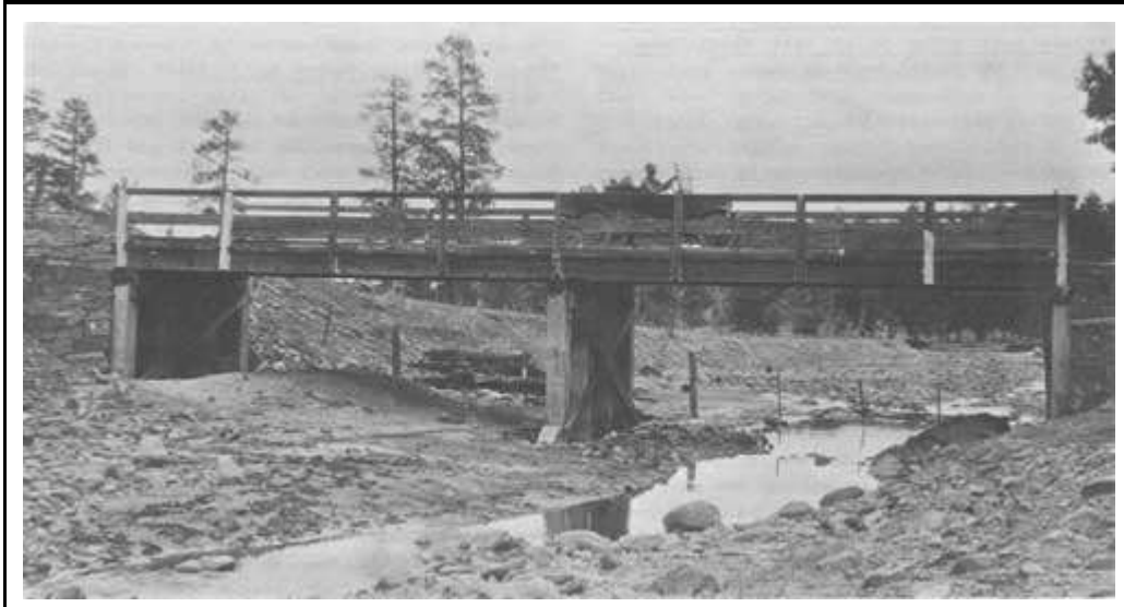
Figure 5. An early-day wooden bridge constructed by the Forest Service.
