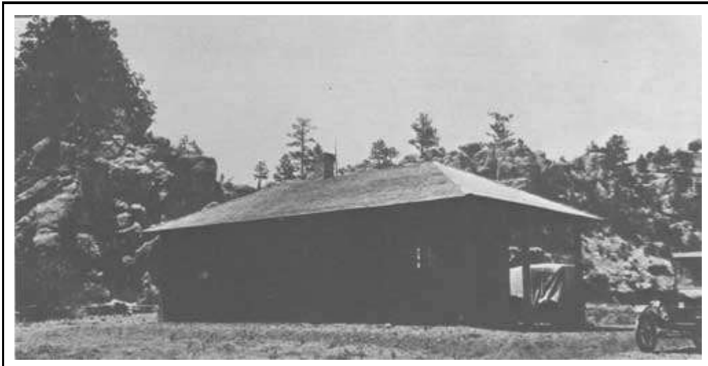
Figure 33. New Beaverhead Ranger Station Datil National Forest June 1923. Photo by John D. Jones
