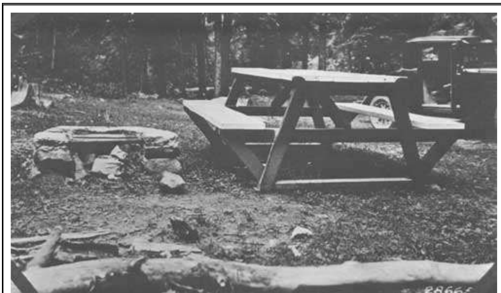
Figure 22. Table and fireplace at Rio Gallinas Campground, Santa Fe National Forest. Built by the Rio Gallinas Civilian Conservation Corp Camp. Photo by John B. Jones, October 1933.
