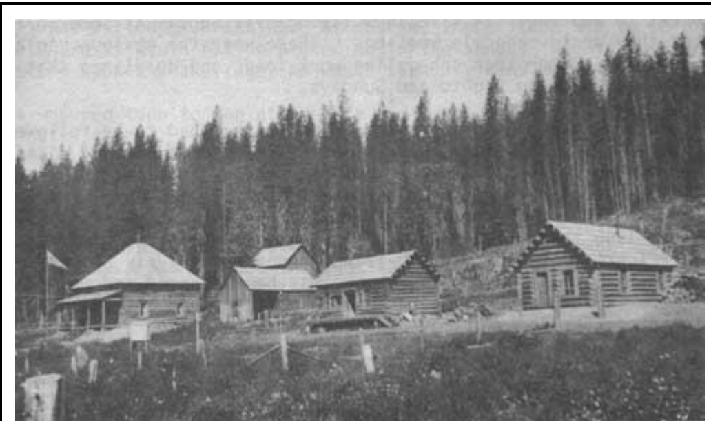
Oxford Ranger Station on Elk Creek, a branch of Orogrande Creek. The structures are similar to others built in the early days of the Forest Service. Photo taken in 1921 or 1922.
