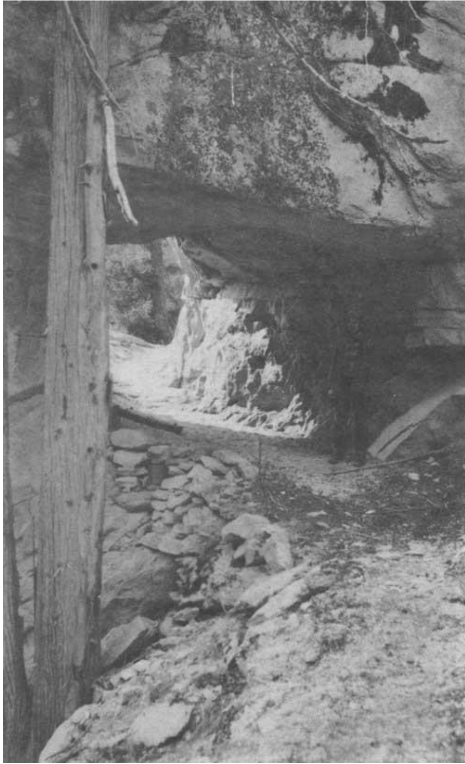
A tunnel along the North Fork trail below Bungalow. Construction of the North Fork Road in 1955 wiped out the tunnel.
