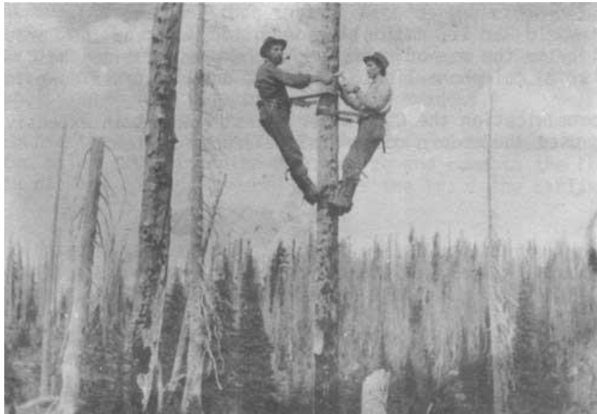
Omer Snyder and Ralph Teed constructing telephone line near Cook Mountain in 1916.
