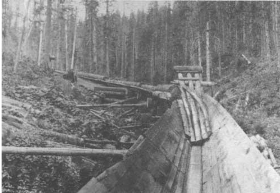
A portion of the old Beaver Creek flume which was used to float logs down the slopes to the North Fork. It was used from 1933 to 1944 until the advent of a more extensive road system ended its usefulness.
