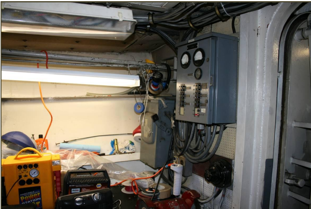
Work bench in engine room in Sitka Ranger, Sitka, Alaska
