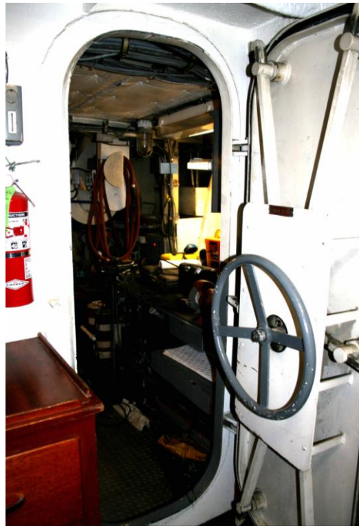
Access to engine room from forecastle looking aft, Sitka Ranger , Sitka, Alaska
