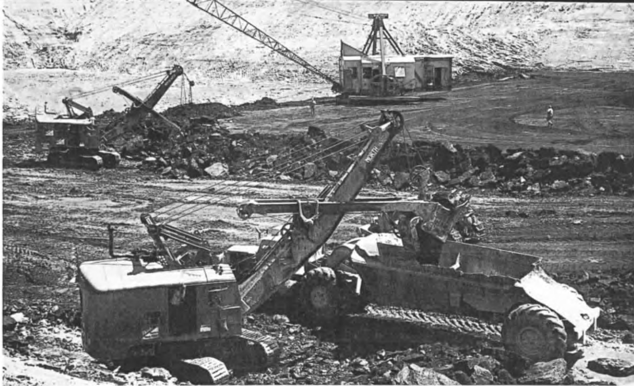
Before North Dakota's Garrison Dam (a Bureau of Reclamation project) was built, this heavy equipment moved in and "rescued" an 11-foot-thick seam of lignite, 750,000 tons, which would have been under water and inaccessible if the dam had been completed before its removal.
