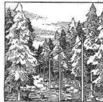
Telephone right-of-way is cleared to avoid contact with trees and branches.
