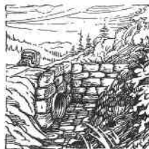
Head wall of culvert.
