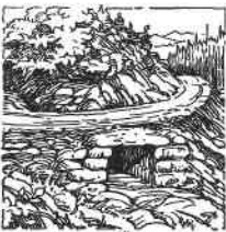
A stone culvert.
