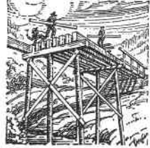
A timber trestle bridge partially completed.
