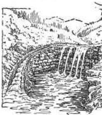
Fish ladder built at dam.
