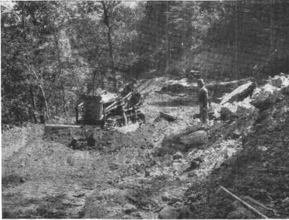
Bulldozers speed up trail construction.
