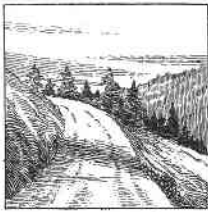
Water will flow over an out-sloped trail.
