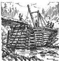
Building a timber crib bridge.
