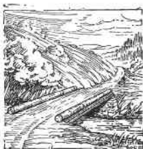
A short span log bridge.
