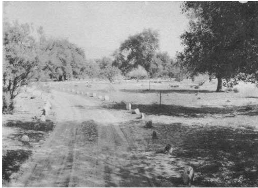
Improper Type of Obstacle A ditch or a fence would be preferable.
