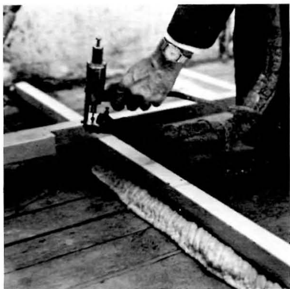
To speed installation of new flooring in urban rehabilitation, a floor-leveling device was developed at the Laboratory at Princeton, West Virginia. New floor screeds are held in place over the old sagging floor, and plastic foam is sprayed under them to hold them in level position and bond them to the old floor.
