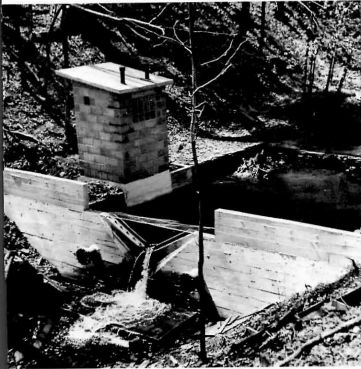
The weir on a gaged watershed on the Fernow Experimental Forest in West Virginia. A continuous record of watershed behavior will show how forestry measures and logging affect the water resource. An automatic recorder in the gage house charts the behavior of the stream.
