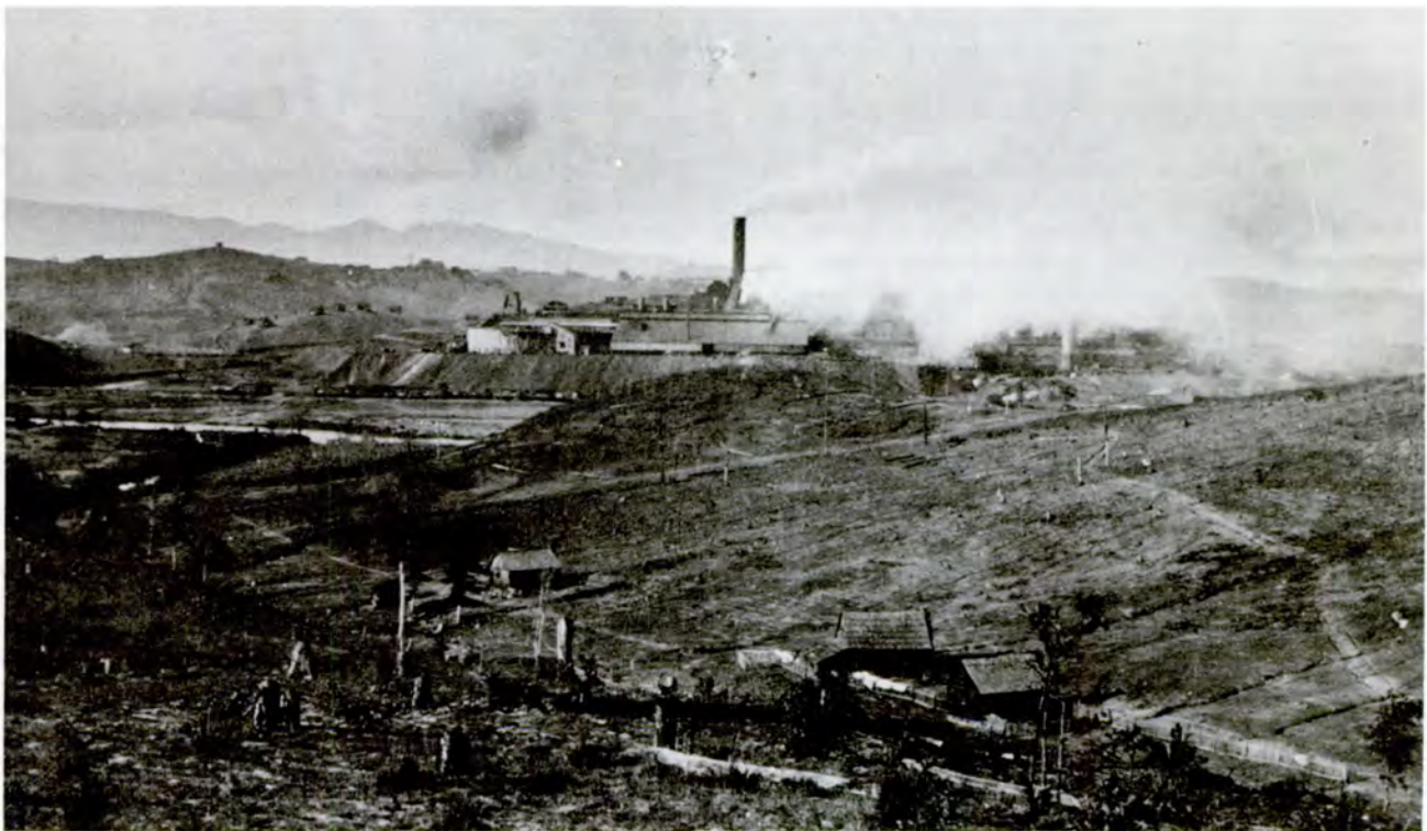
Figure 14.—Smelter of Tennessee Copper Company at Copper Hill-McCaysville on Tennessee-Georgia State line in Southern Appalachian Highlands along Ocoee River. When photo was taken in September 1905, plant was undergoing great expansion. Forest devastation from sulfur fumes of smokestacks was already evident. Area is near the edges of three National Forests and three States. Acid fumes from this and other smelters in the “Copper Basin” destroyed timber and wildlife on thousands of acres of forests and caused severe soil erosion for many years, muddying waters of the Tennessee River, more than 40 miles distant, before operations ceased. (NA:95G-63040)
