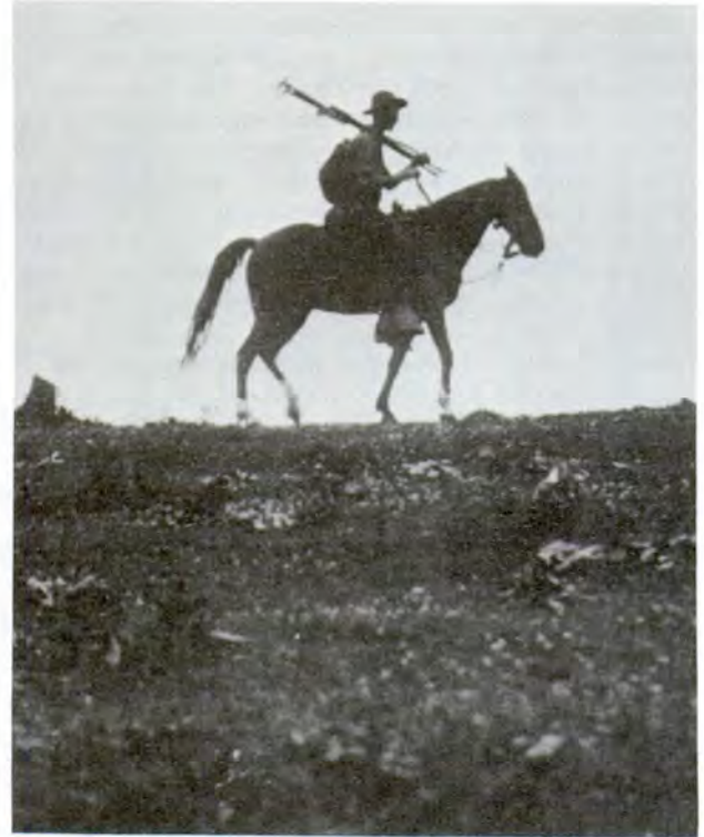
Figure 34.—Pisgah National Forest officer using a portable telephone hooked up to a newly installed Forest Service field line. Note wire hanging down from the overhead wire strung through the woods. The Pisgah was still a Purchase Unit when photo was taken in April 1916; it was officially established as the first purchased National Forest in the United States in October 1916. (NA:95G-27361A)
