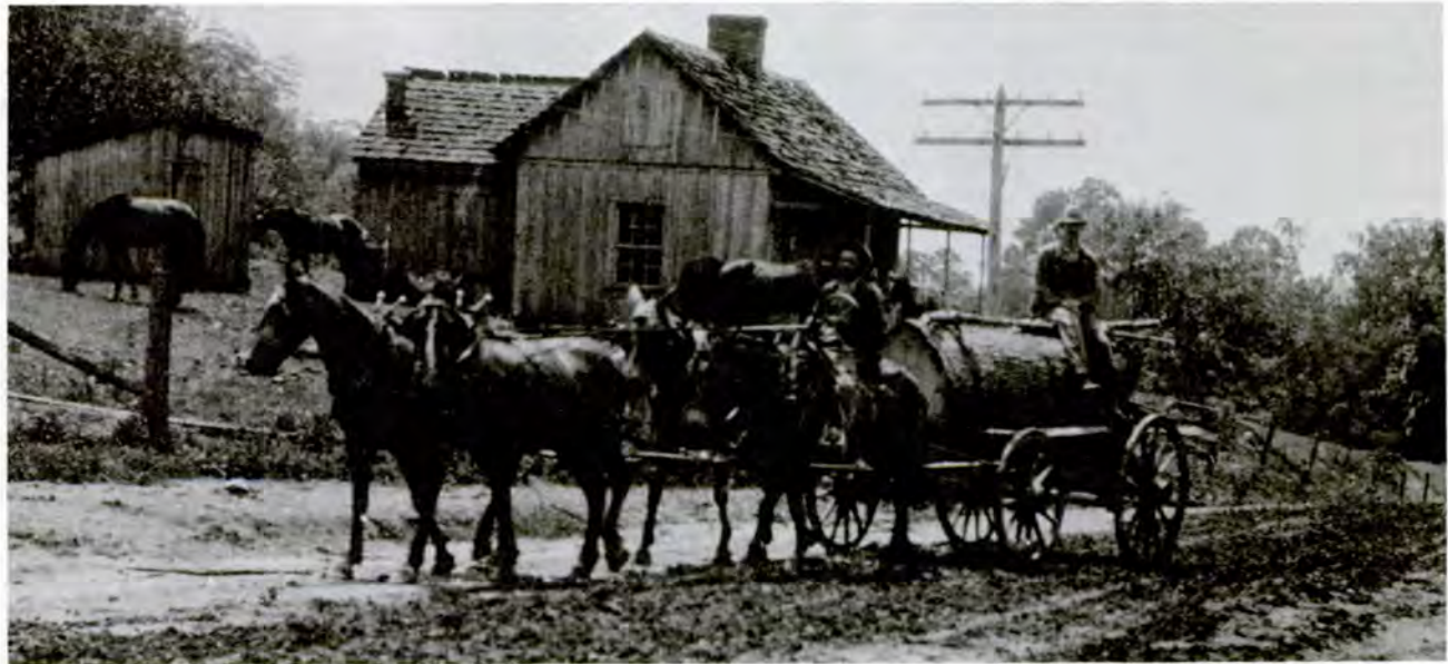
Figure 11.—A team of four horses and mules pulling a flatbed wagon carrying a large white oak log to the sawmill along a dirt road near Jonesboro, Washington County, Tenn., in July 1915. Log probably came from Locust Mountain area west of Johnson City, not far from the Unaka National Forest, now a part of the Cherokee. (NA:95G-23262A)
