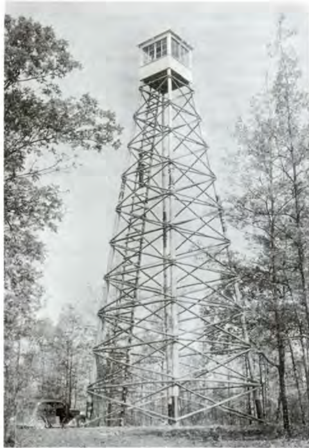
Figure 70.—Beulah Heights fire tower, a temporary structure of southern yellow pine with a 7- x 7-foot cabin, built by Civilian Conservation Corps enrollees. Daniel Boone (then Cumberland) National Forest, Ky., shown in April 1938. (National Archives: Record Group 95G-365411)
