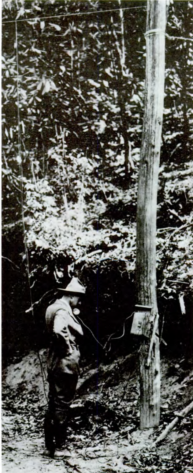
Figure 34.—Pisgah National Forest officer using a portable telephone hooked up to a newly installed Forest Service field line. Note wire hanging down from the overhead wire strung through the woods. The Pisgah was still a Purchase Unit when photo was taken in April 1916; it was officially established as the first purchased National Forest in the United States in October 1916. (NA:95G-27361A)
