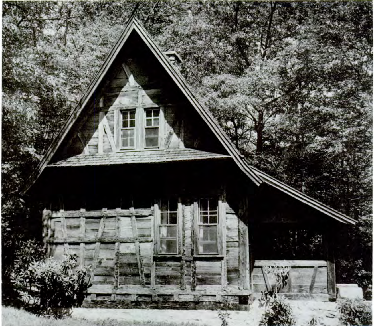
Figure 20.—Schenck Lodge, built in Black-Forest-of-Germany style on site of old Biltmore Forest School, now the Cradle of Forestry Visitors Center, Pisgah National Forest, Brevard, N.C., as it appeared in August 1949. Lodge had just been restored with new roof and foundation. It was originally built to house forest workers on the old Biltmore Forest, and then to house students in Dr. Carl A. Schenck's school. It is now used for administration and public recreation. (Forest Service photo F-458641)
