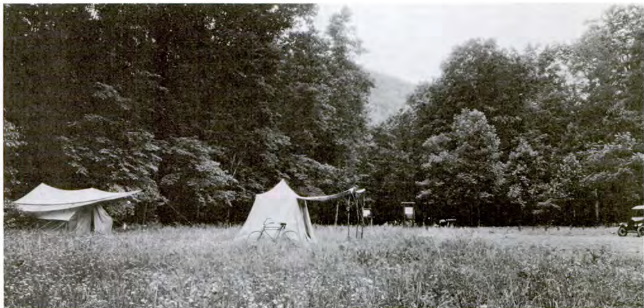
Figure 56.—Bent Creek Forest Camp, overnight public recreation site on Pisgah National Forest near Asheville, N.C., in March 1930. (NA:95G-238168)
