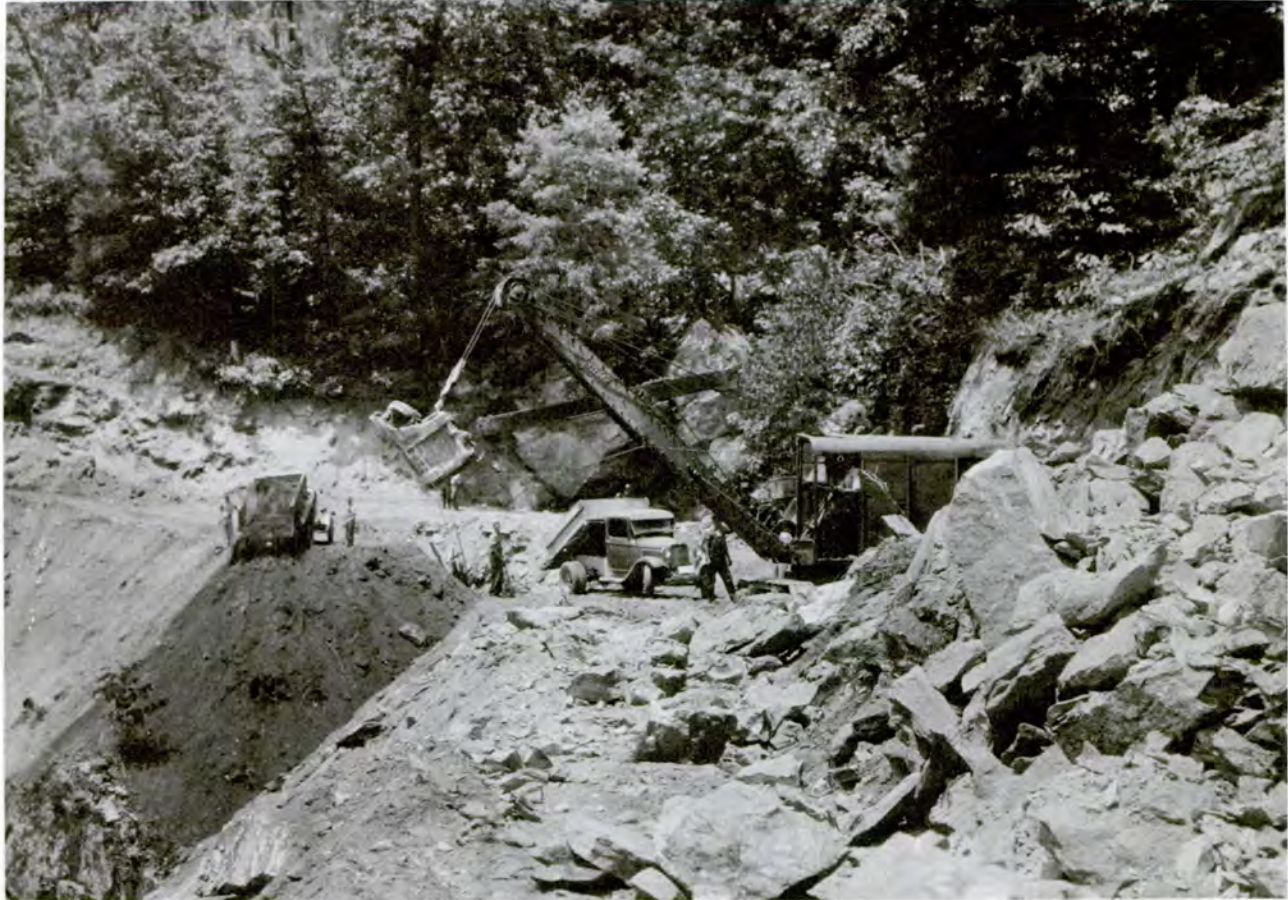
Figure 51.—Construction work on State Route 106 on Scaly Mountain between Highlands, N.C., and Dillard, Ga., in summer 1937. Job was done under the Federal Emergency Relief Administration (ERA), which became the Works Progress Administration (WPA) in 1938. (NA:95G-352573)
