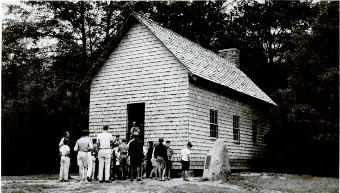
Figure 21.—Replica of original Biltmore Forest School building on Pisgah National Forest, Brevard, N.C., south of Asheville, now part of the Forest Service's Cradle of Forestry Visitor Center. Photo was taken in August 1967, a year after reconstruction. (Forest Service photo F-516882)
