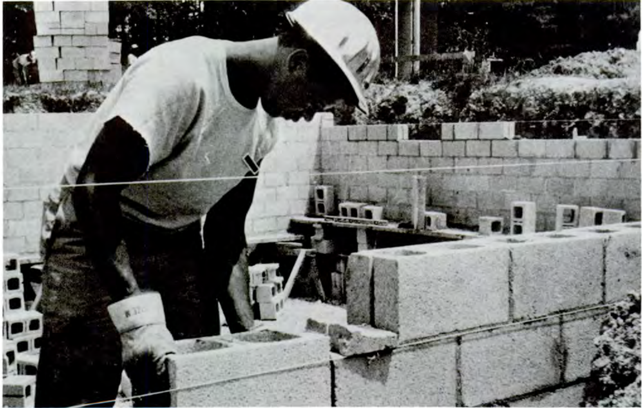
Figure 104.—Cinder blocks for new office building of Stanton (formerly Red River) Ranger District being laid by Job Corps trainee in June 1967. The men on this project were from the Frenchburg Civilian Conservation Center, near the Red River Gorge and the confluence of Menifee, Powell, and Wolfe counties, on the Daniel Boone National Forest, Ky. (Forest Service photo F-519122)
