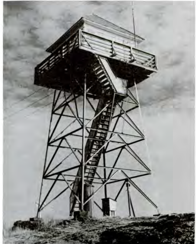
Figure 92.—Steel lookout tower on Black Mountain near Woody Gap, Suches, Ga., on Chattahoochee National Forest, December 1952. Chestatee (formerly Blue Ridge) Ranger District. (Forest Service photo F-470980)
