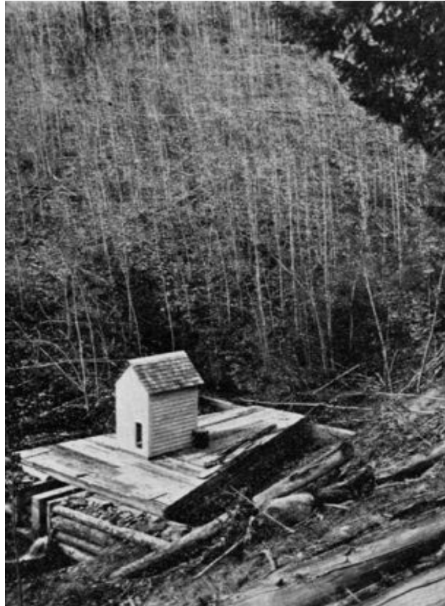
Image 6: The evaluation station at the Wagon Wheel Gap Project in Colorado. This was the model for later small forest watershed studies in the U.S. with a control watershed and an observation period prior to treatment. Photo from the USDA Weather Bureau (1928).
