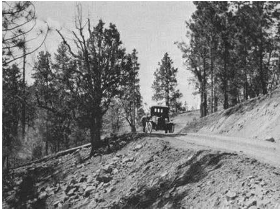
Road between Alpine, Arizona, and Luna, New Mexico, May 1924.
