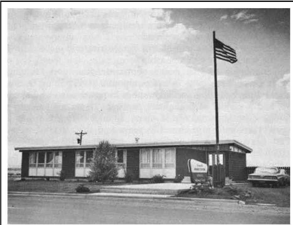
A modern District Forest Ranger's Office, Springerville, Apache National Forest.
