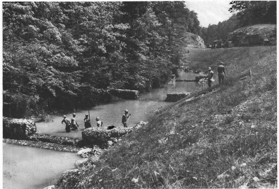
Job Corps enrollees building gabions for stream improvement and watershed protection on the Middle Fork of the Red River, Daniel Boone National Forest, Kentucky.
