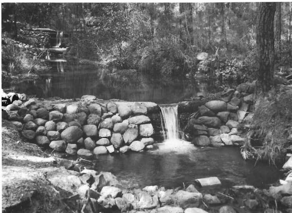
Fish dams on stream in Poliza Canyon on the Santa Fe National Forest, New Mexico, 1936. These dams benefit fish, wildlife, riparian area, stream channel condition, and stream condition and flow.
