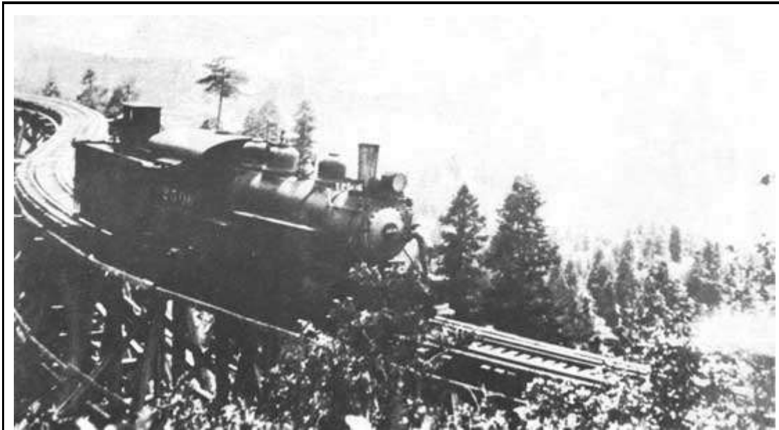
Figure 48. SP 2506 standing on the "S" trestle below Cloudcroft, ca. 1936. ( E. Clack collection )
