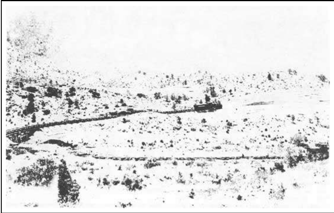
Figure 40. In early 1902, the brand new Shay patent geared locomotive, number 105, pulled a 334-ton train of 41 empty log cars from Alamogordo to Toboggan. The train was stopped for the photographer on the "S" curve between El Valle and Pinto. ( Baldwin-Lima-Hamilton Corp. collection )
