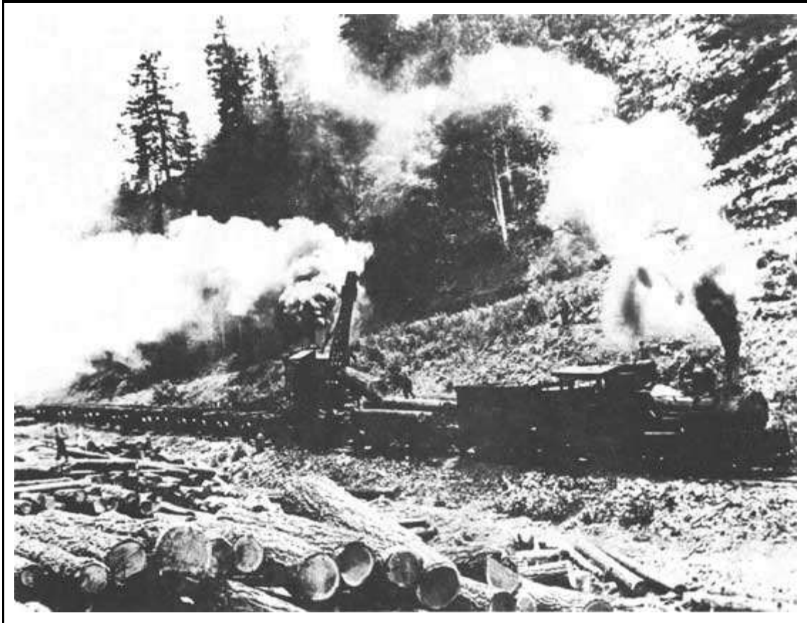
Figure 42. Southwest Lumber Company loading logs in Water Canyon. Shay locomotive number 6. June 28, 1928. (By E. S. Shipp. USDA Forest Service photo 233024)
