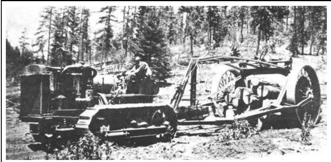
Figure 20. Caterpillar tractor and hydraulic arch hauling logs for George E. Breece Lumber Co. on Mescalero Apache Reservation. (By J. D. Jones, USDA Forest Service photo 230661)
