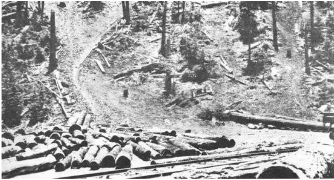
Figure 52. Log chute or skidway in action, with boy "greasing the skids." June 26, 1928. (By E. S. Shipp. USDA Forest Service photo 233058)
