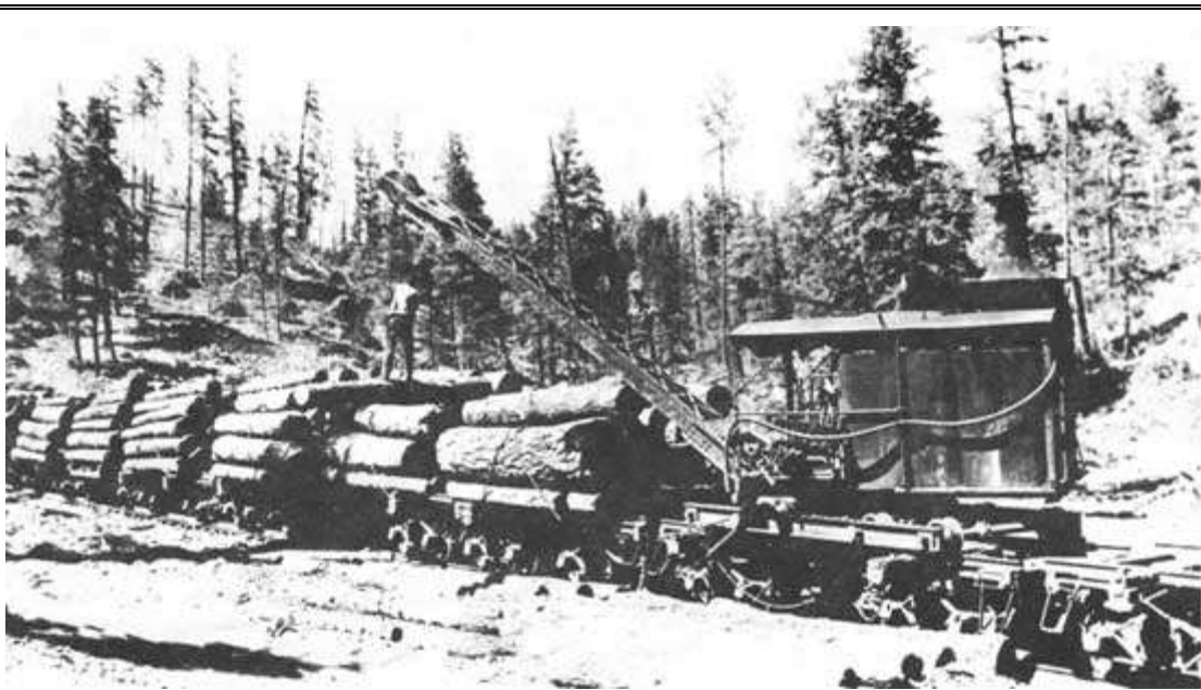
Figure 32. George E. Brece Lumber Co. loader working at landing on Mescalero Apache Reservation. The loader moves from car to car on rails permanently mounted on each car. June 30, 1928. (By E. S. Shipp . USDA Forest Service photo 233085 )
