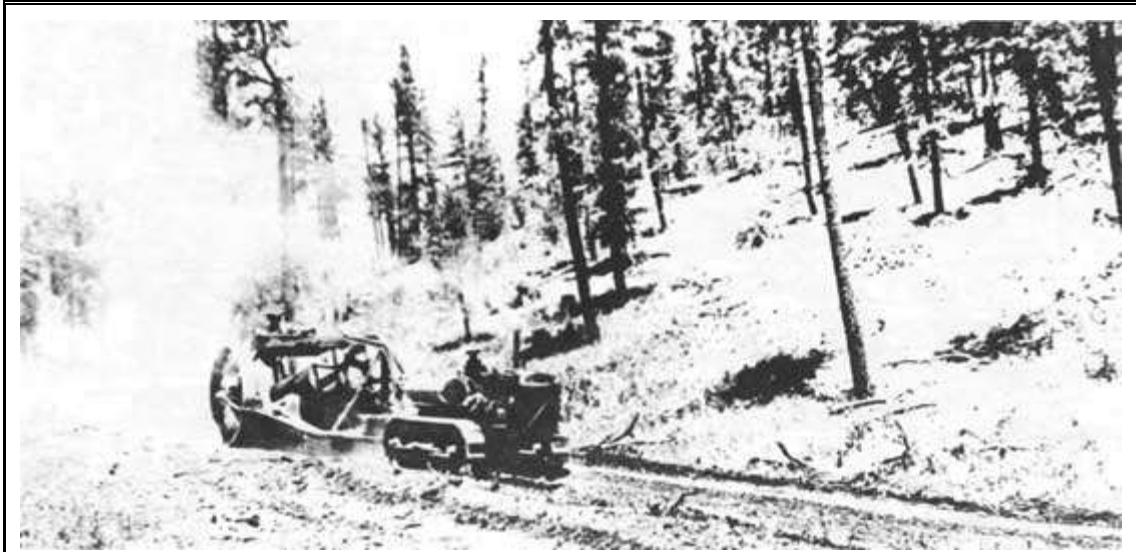
Figure 30. Skidding logs with hydraulic arch and Caterpillar tractor on the Mescalero Apache Reservation. George E. Breece Lumber Co. June 30, 1928. (By E. S. Shipp. USDA Forest Service photo 233084)
