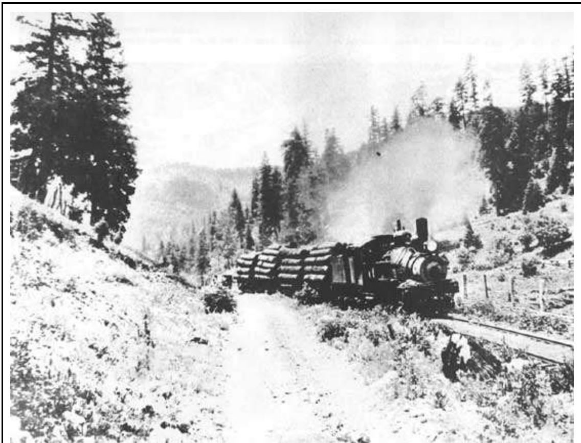
Figure 41. Southwest Lumber Company log train near Russia hauled by Shay locomotive number 1. June 27, 1928. (By E. S. Shipp. USDA Forest Service photo 233046)
