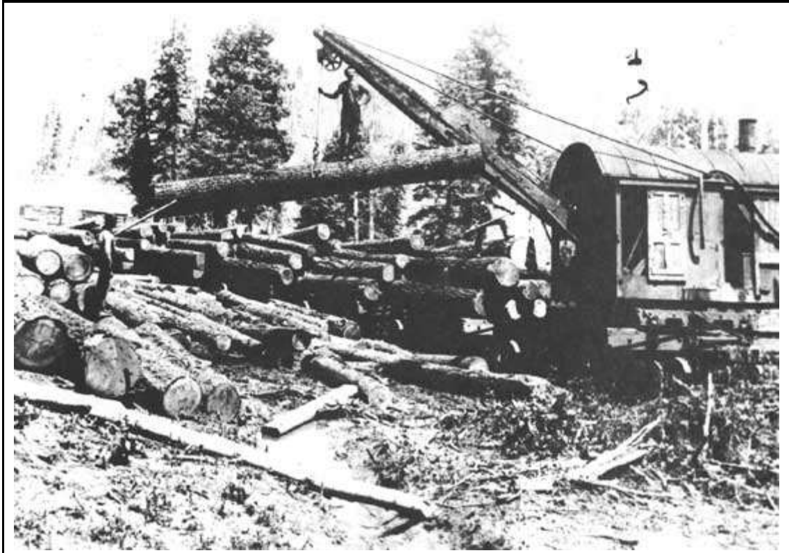
Figure 10. Alamogordo Lumber company steam log loader at work ca. 1889. (By Green Edward Miller. Museum of New Mexico)
