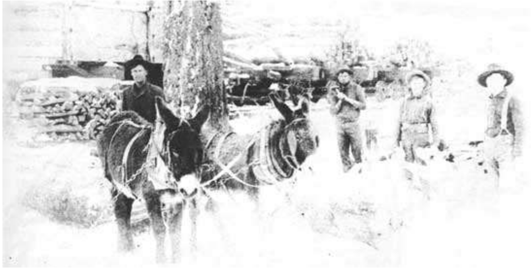
Figure 54. Mule team skidding logs in winter on the Almagordo Lumber Company. The log cars behind the team are loaded with ties and, on the left, a primitive water tank. n.d. (By Green Edward Miller. Museum of New Mexico Collection)
