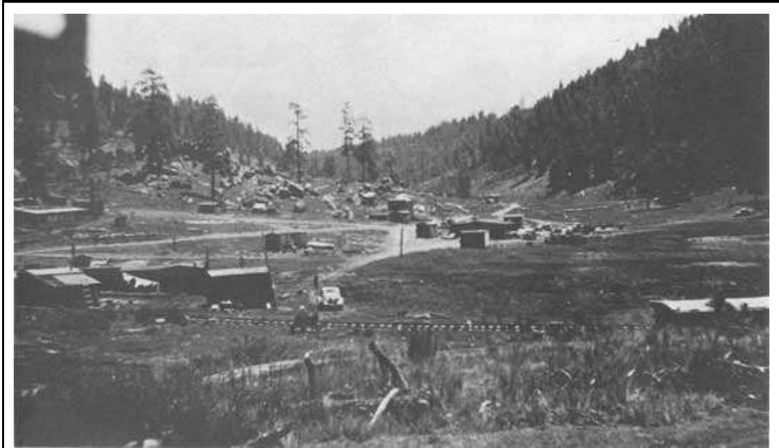
Figure 40. Ojitos camp circa 1937 - 1939. Living quarters are in the left foreground, railroad spur running across, and the truck shop is center right to the rear. ( Photo by Yale Weinstein )
