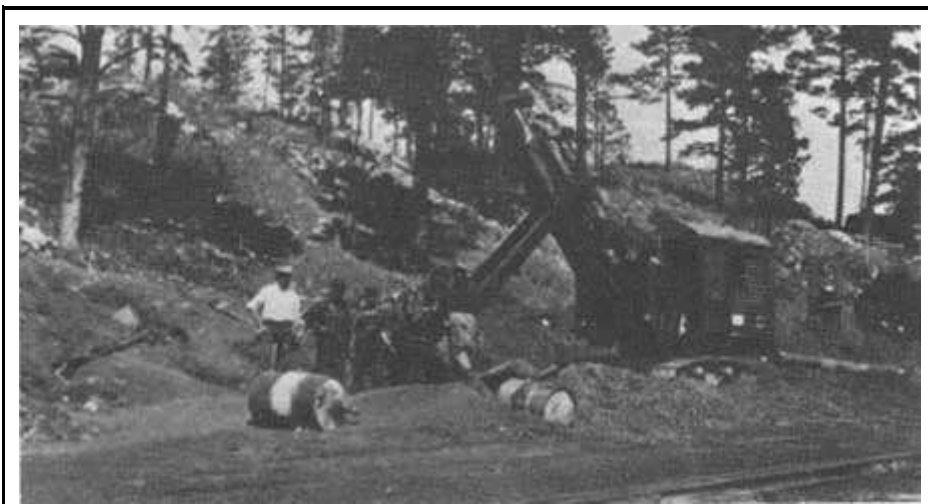
Figure 29. This power shovel on a tracked chassis was used for road building circa 1932. The use of power machinery greatly speeded the work of transporting logs from the woods. (From the collection of T. P. Gallagher, Jr.)
