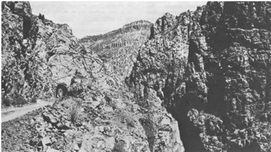
Figure 63. The approach to the first tunnel in Guadalupe Box, The road seen on the left is directly on the old railroad bed. This view was photographed on August 21, 1960, by Henry E. Bender, Jr.
