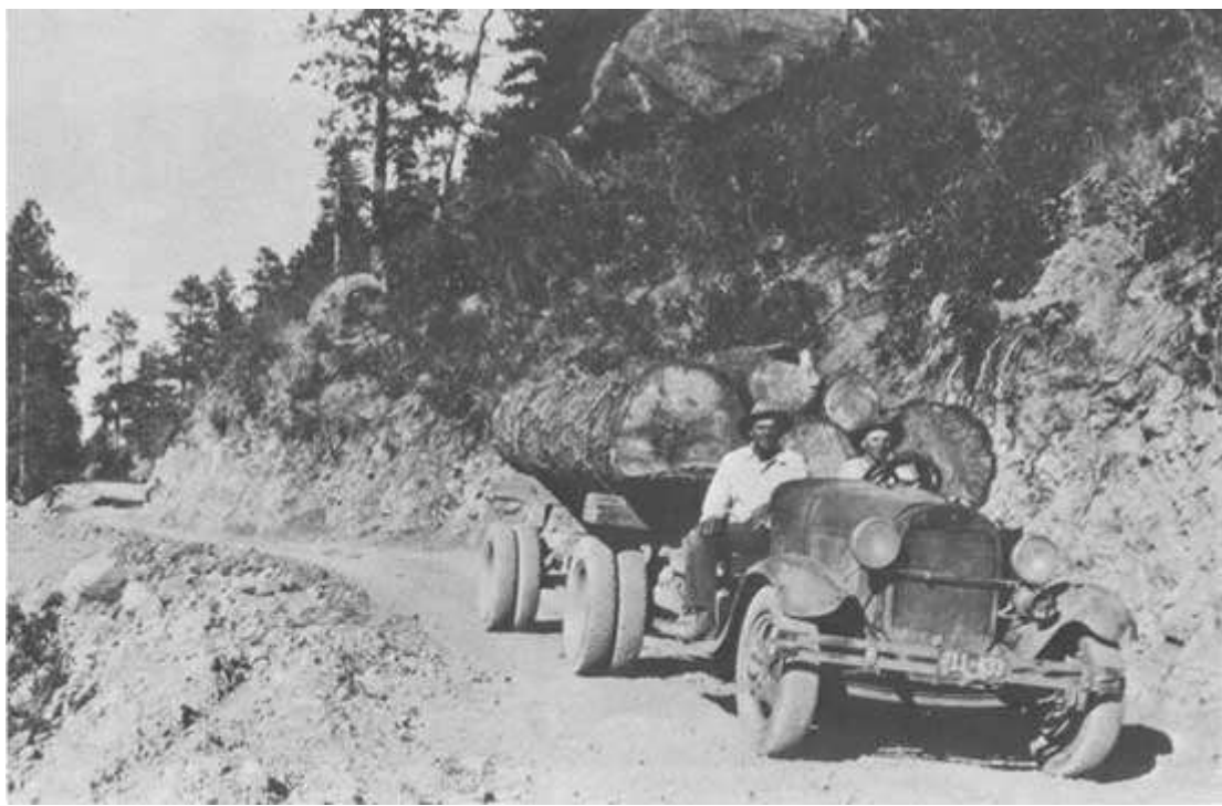
Figure 42. A detailed view of one of the early log trucks, circa 1932. In most respects, this rig shows the same design features -- articulated trailer, dual tires, and wide log bunks -- that characterized later and heavier trucks. Provisions for the drivers safety and comfort, however, left something to be desired. (From the collection of T. P. Gallagher, Jr.)
