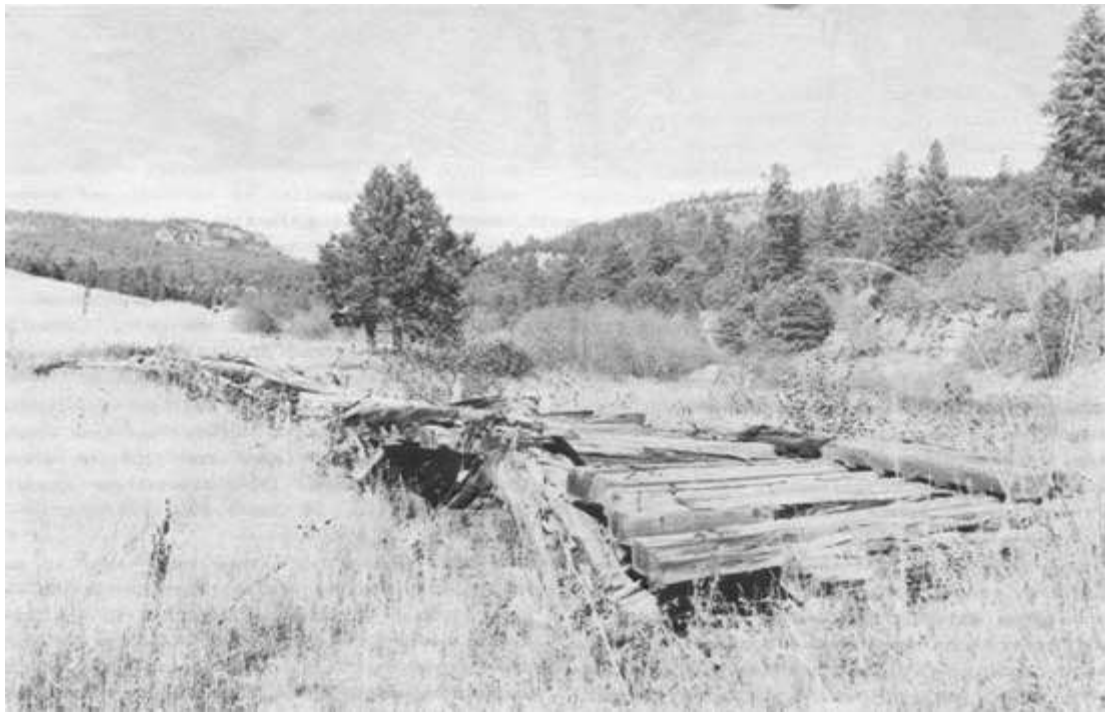
Figure 37. The railroad trestles along the Rio de las Vacas north of Porter were characterized by long log stringers and cribwork supports. Most were very low and vulnerable to washouts. This view shows such a bridge in November, 1968, some 27 years after abandonment of the railroad. ( Photo by Vernon J. Glover )
