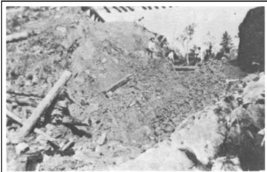
Figure 30. A large washout of a timber trestle circa 1932. Nearly the entire structure has disappeared, leaving the track swinging across the gully. ( From the collection of T. P. Gallagher. )
