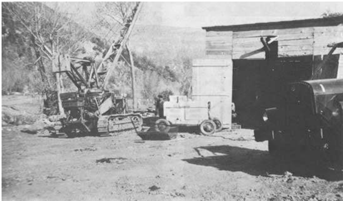
Figure 80. The truck repair shop at O'Neil landing circa 1939. Equipment (from left to right) is the Bucyrus-Erie Loadmaster, a Lincoln electric welder, and the nose of the Kenworth diesel log truck Number 1. (Photo by Yale Weinstein)
