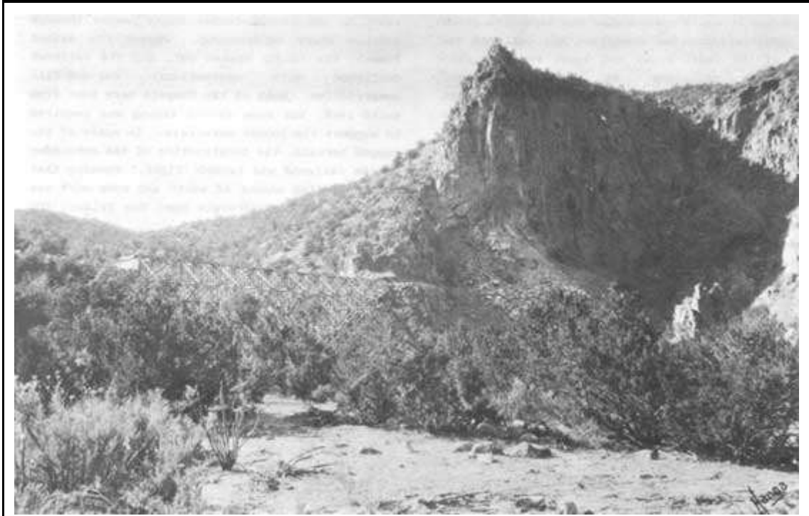
Figure 9. The southern approach to the Guadalupe Box, showing the fills and the high trestle required to reach the tunnels. The roadbed was climbing steadily throughout this section. ( Photo by M. E. Hanna. Albuquerque Public Library collection )
