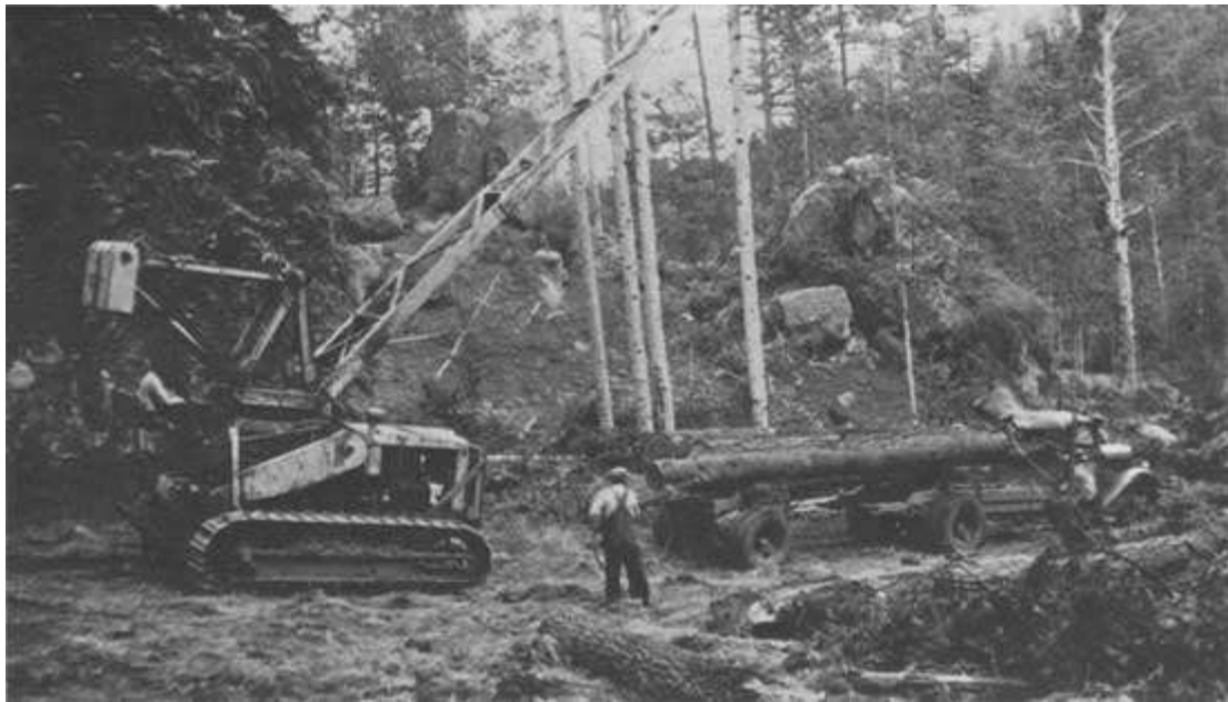
Figure 92. A Bucyrus-Erie Loadmaster at work in the woods, circa 1937 - 1941. This machine combined the features of a Caterpillar tractor and a power crane in one unit capable of lifting, moving, and loading logs efficiently. The boom was capable of rotating as well as lifting, although the lack of outriggers must have severely limited its capacity while positioned to the sides. (Photo by Yale Weinstein)
