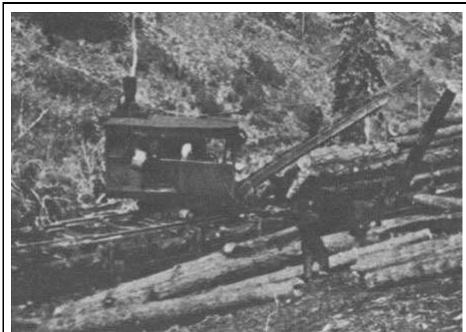
Figure 3. American Hoist & Derrick Company log loader lifting logs onto railroad cars, circa 1932. The sets of rails on which the loader moved itself from car to car are seen on the left. Following each move the loader picked up the set of rails it had just vacated and swung it into place ahead. (Photo from T. P. Gallagher, Jr., collection)
