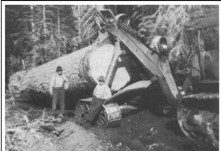
Figure 94. A Caterpillar tractor skidding a very large log with a Hyster steel arch, also on tracked wheels, This view, from the C. O. Clark collection, probably dates from the 1930s.
