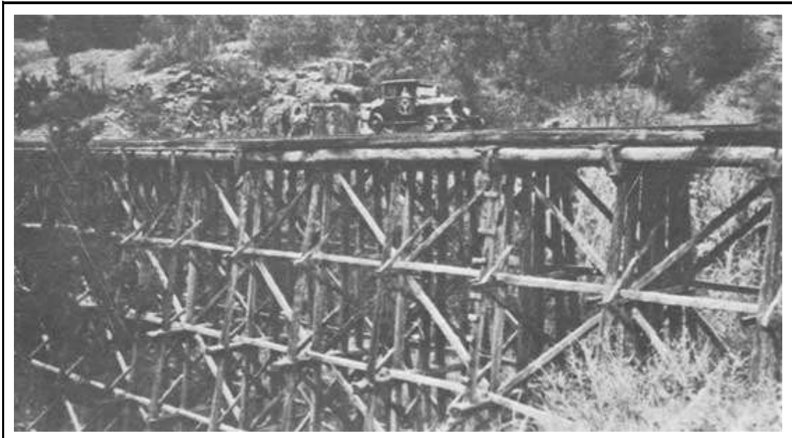
Figure 43. A "rail-auto" as it was termed on the Santa Fe Northwestern Railway, posed on a tall trestle circa 1932. This construction was typical of the railroad line along the Rio Guadalupe between the Box and Porter. This trestle was of typical railroad design except for the use of long logs as stringers under the ties instead of the usual milled timbers. ( Photo from the collection of T. P. Gallagher, Jr. )
