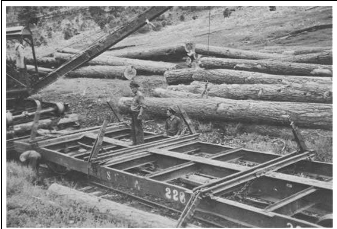
Figure 11. A steel log car of the SFNW in the summer of 1939 at O'Neil Landing. The structure of the car and the design of the log bunks and folding stakes are clearly shown. ( Photo by Yale Weinstein )
