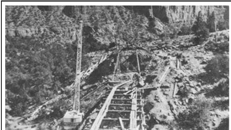
Figure 48. View from the track approach to the Joaquin Canyon trestle construction in the autumn of 1939. The track level on the opposite side of the canyon is seen above the hoist posts at the far end of the trestle. Riprap protects the embankment. (Photo by Yale Weinstein)
