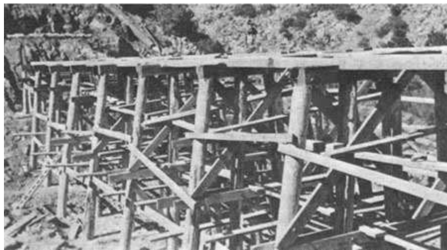
Figure 47. Details of typical railroad trestle construction are seen in this view of the Joaquin Canyon bridge. The vertical piles carried the load and the many braces, both lateral and longitudinal, provided stability under the moving loads of heavy trains. (Photo by Yale Weinstein)
