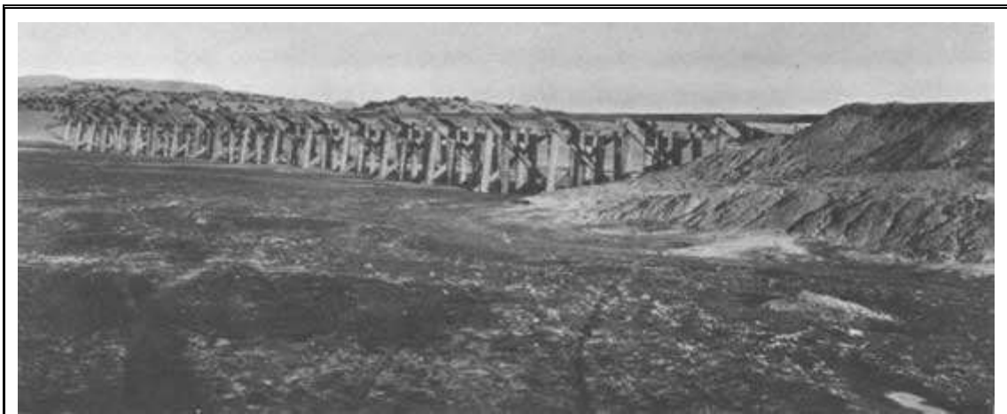
Figure 6. Typical low pile trestle crossing an arroyo circa 1923. (Photo by M. E. Hanna. Albuquerque Public Library collection)
