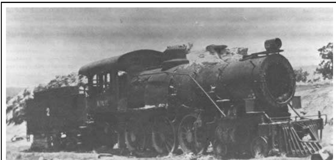
Figure 61. Abandoned hulk of San Juan Coal & Coke Company locomotive Number 2, circa 1938, near La Ventana.
