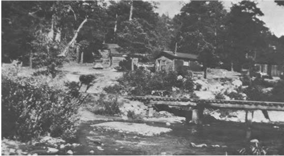
Figure 16. A railroad trestle and dwellings scattered through the woods at Porter, New Mexico, circa 1932. (Photo by Don R. Hammond)
