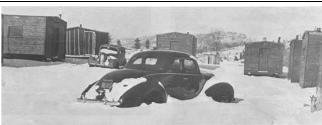
Figure 70. Bachelor quarters at O'Neil Landing during the winter shutdown, circa 1939. It looks as if the roads were closed. (Photo by Yale Weinstein)
