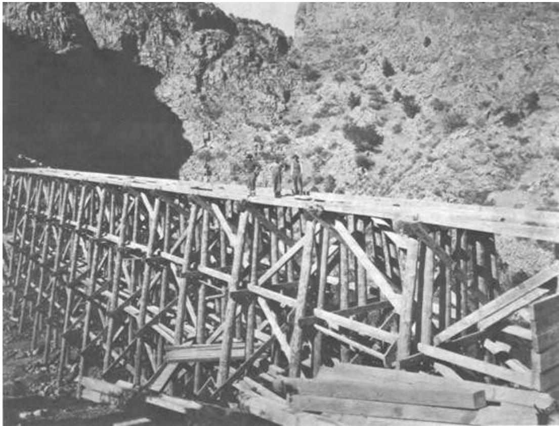
Figure 8. The large trestle leading to the Guadalupe Box tunnels during construction, circa 1924. Many features of trestle construction are shown in this view. Note the six piles in each bent, and the numerous horizontal and diagonal braces. The heavy stringers or longitudinal members to support the crossties were being installed at this time. ( Photo by M. E. Hanna. Albuquerque Public Library collection )
