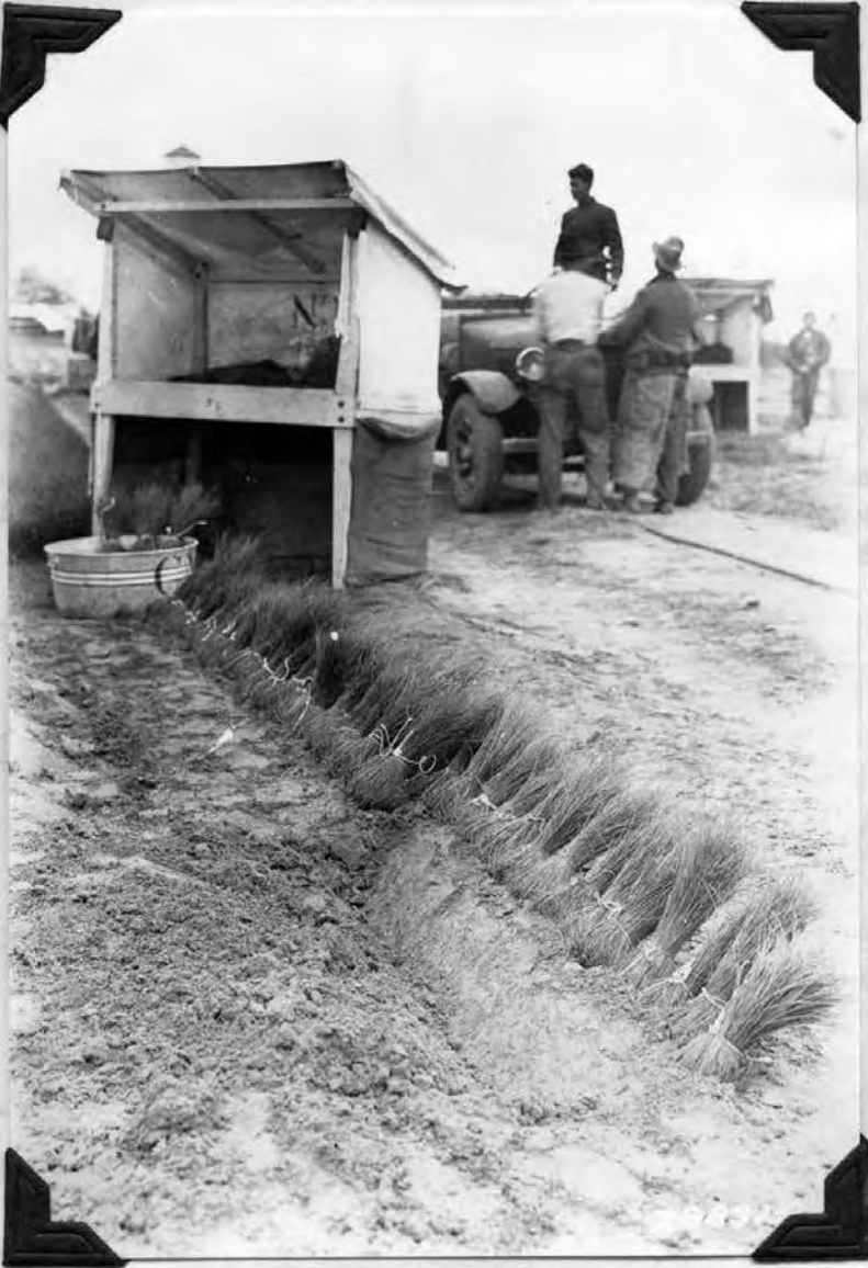
Heel-in trench, showing the sloping face and heeled-in longleaf bundles.
