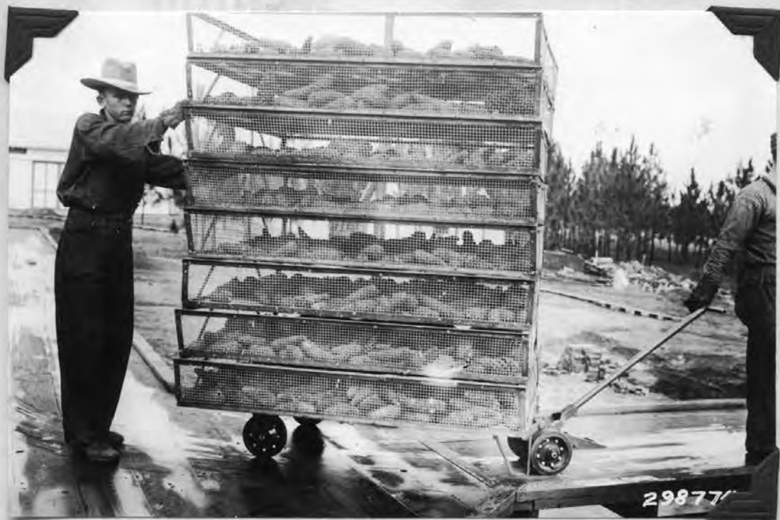
Wheeling the loaded cone trays from the curing sheds to the extractory.
