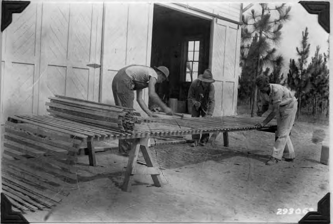
Constructing lath shades.
