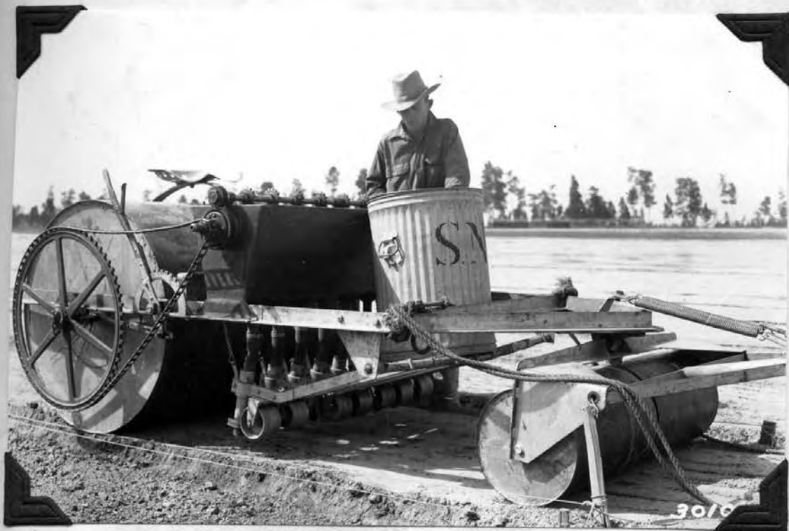
Williamson longleaf drill seeder, developed at the Stuart Nursery as a modification of the Hazard drill seeder.
