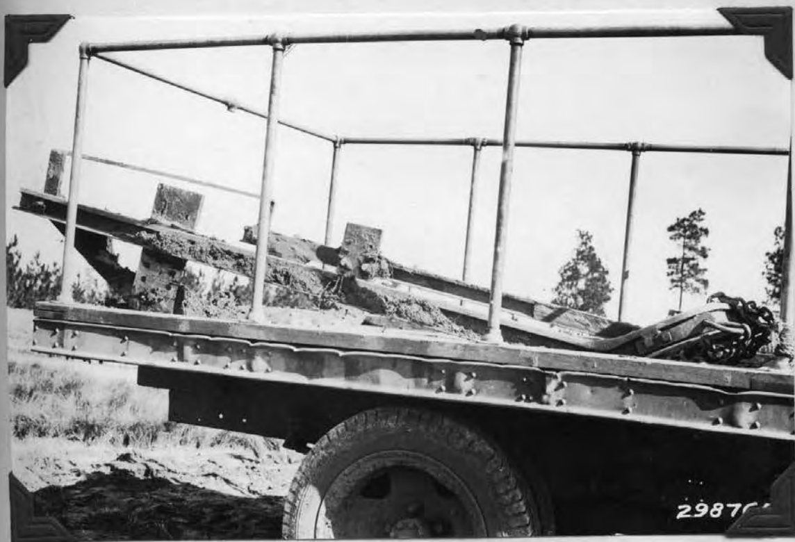
A view of the lifter showing the blade and bracing; placed on a truck for transporting to another part of the nursery.
