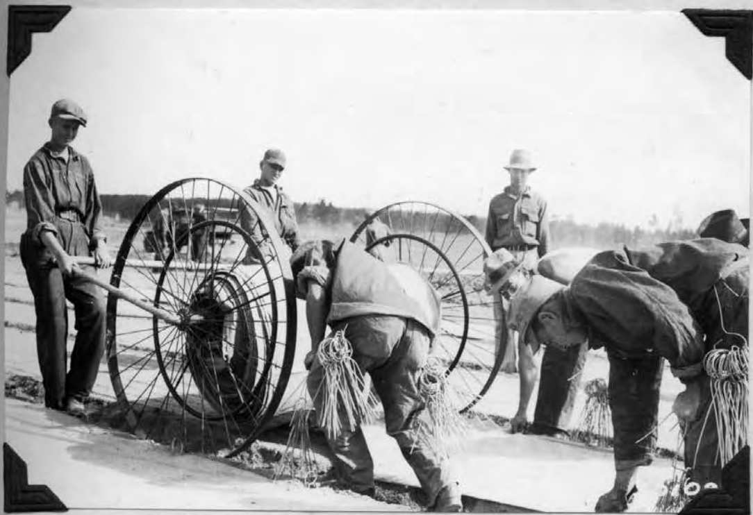
Putting burlap in place and pinning it down.
