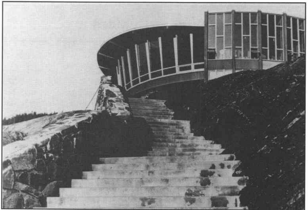
Figure 2-108. The first Forest Service visitor center at Mendenhall Glacier, Juneau, Alaska (1961)
