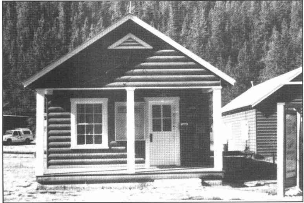
Figure 1-34. Warren Guard Station, Payette National Forest, Region 4 (1934)
