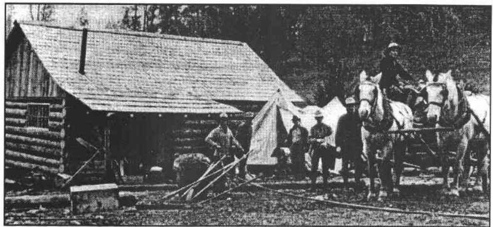
Figure 1-6. Rangers on the Sierra National Forest construct the Jerseydale Ranger Station in the early 1900's. Dolly and Dick, the Reserve's work horses, assisted.
