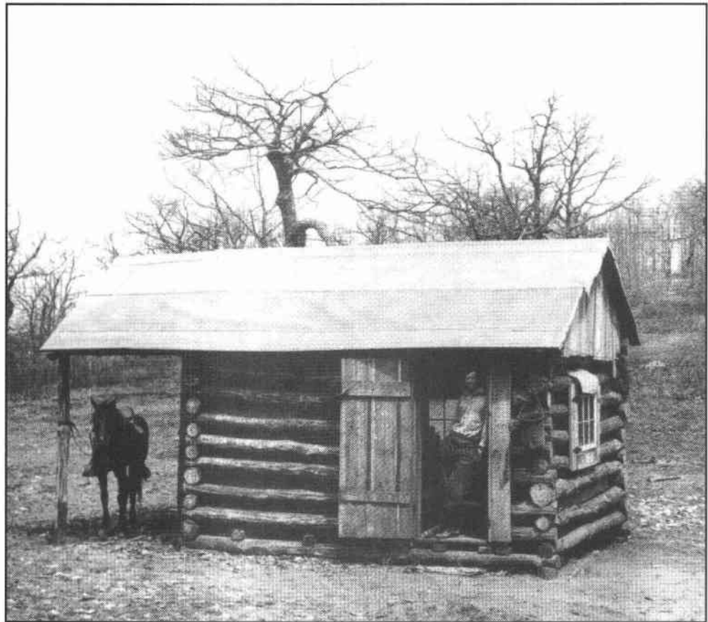
Figure 1-4. Log shack used as a temporary camp near Silers Bald, Wayah Ranger District, Nantahala National Forest, North Carolina (1916)
