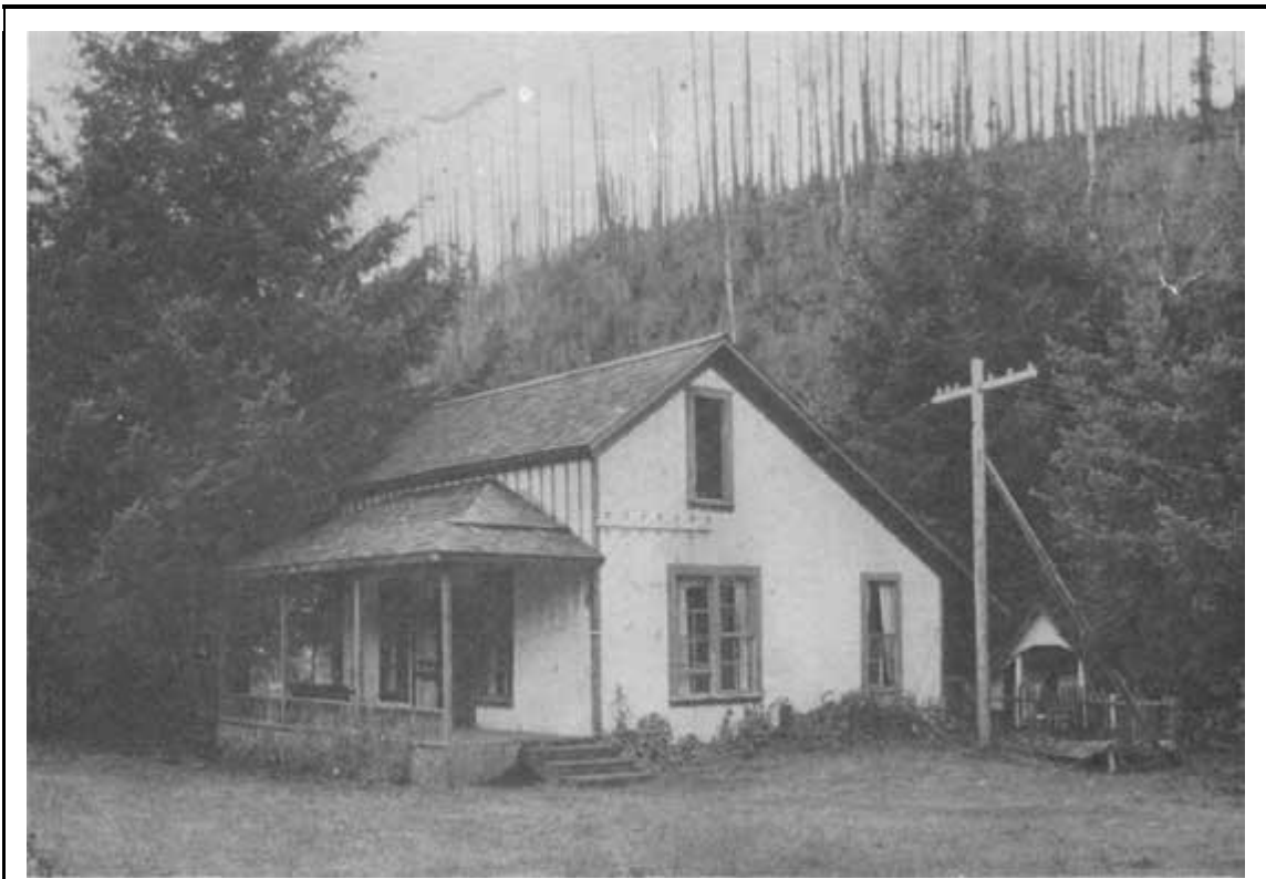
Detroit Ranger Station, c. 1915.
