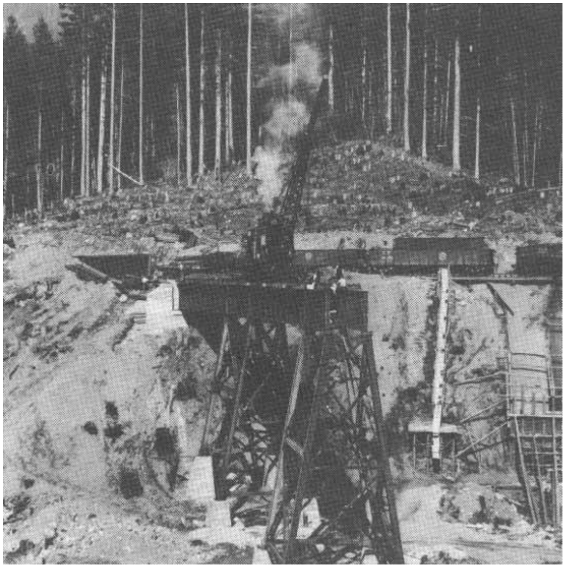
Salt Creek Railroad Bridge, under construction, 1926.
