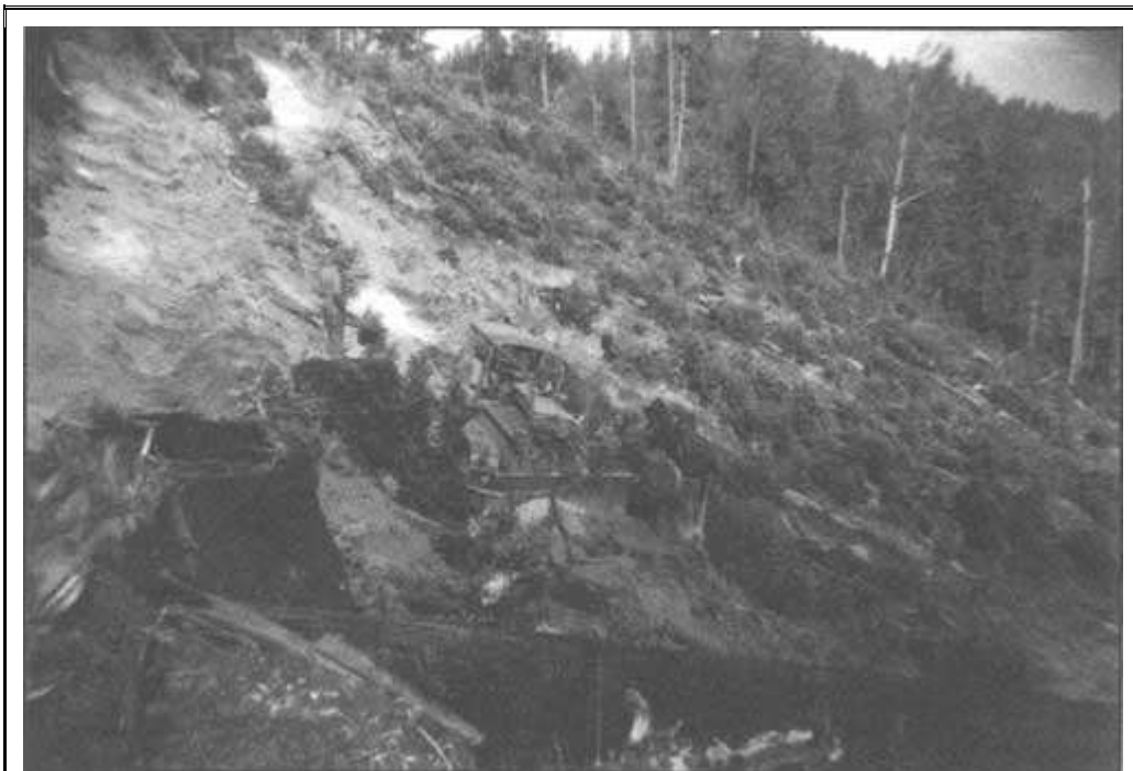
This photo, taken in 1960, shows a D-8 tractor building terraces as a hedge against erosion prior to restocking with trees. This was on the Leary Creek Sale, Orleans Ranger District. US Forest Service photo
