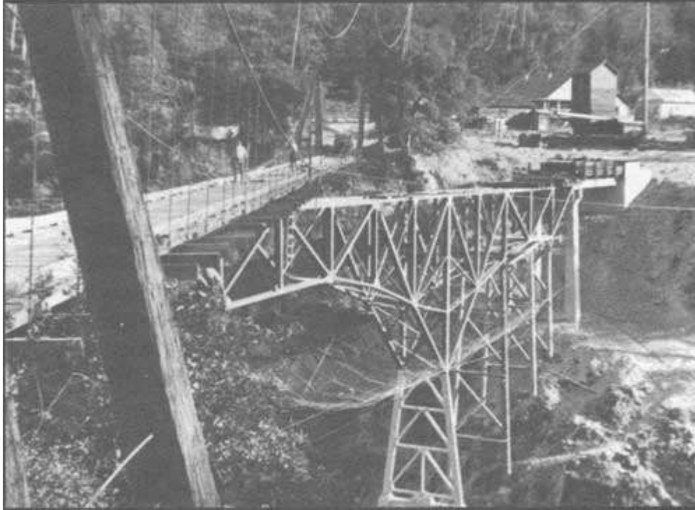
This 1937 photograph shows the Civilian Conservation Corps' construction of the Salyer Bridge. Aimed south, note the old suspension bridge still in place and the safety net below the new bridge. Courtesy of Robert Albrecht
