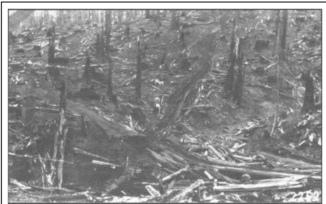
This steam donkey set at a redwood harvest operation graphically shows the aftermath of this destructive yarding method and of the effects of post-harvest intensive burning. This photograph was probably taken in the 1920s. US
