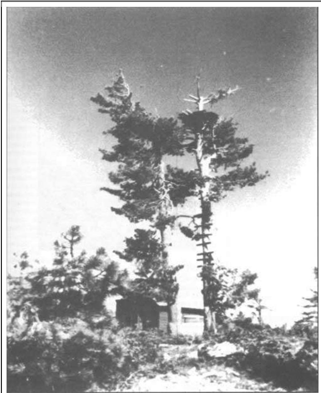
Blue Creek Mountain crow's nest and cabin, Orleans Ranger District. Crow's nests preceded more formal lookout structures. This photo was taken during World War II when Blue Creek Mountain was being used as an Air Warning Service lookout. This lookout no longer exists. US Forest Service photo
