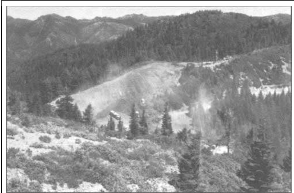
Construction work on the Gasquet to Orleans Road. US Forest Service photo
