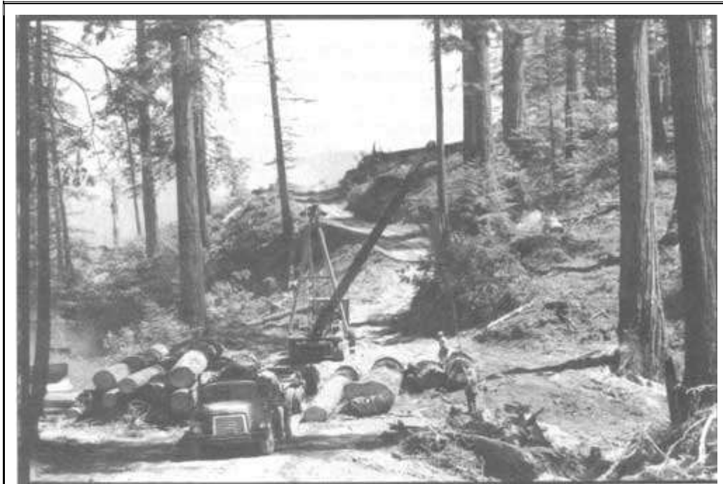
This photograph, probably taken during the 1950s, shows a truck being loaded with old growth Douglas fir. A tractor is working, at the far left, by the log deck. US Forest Service photo
