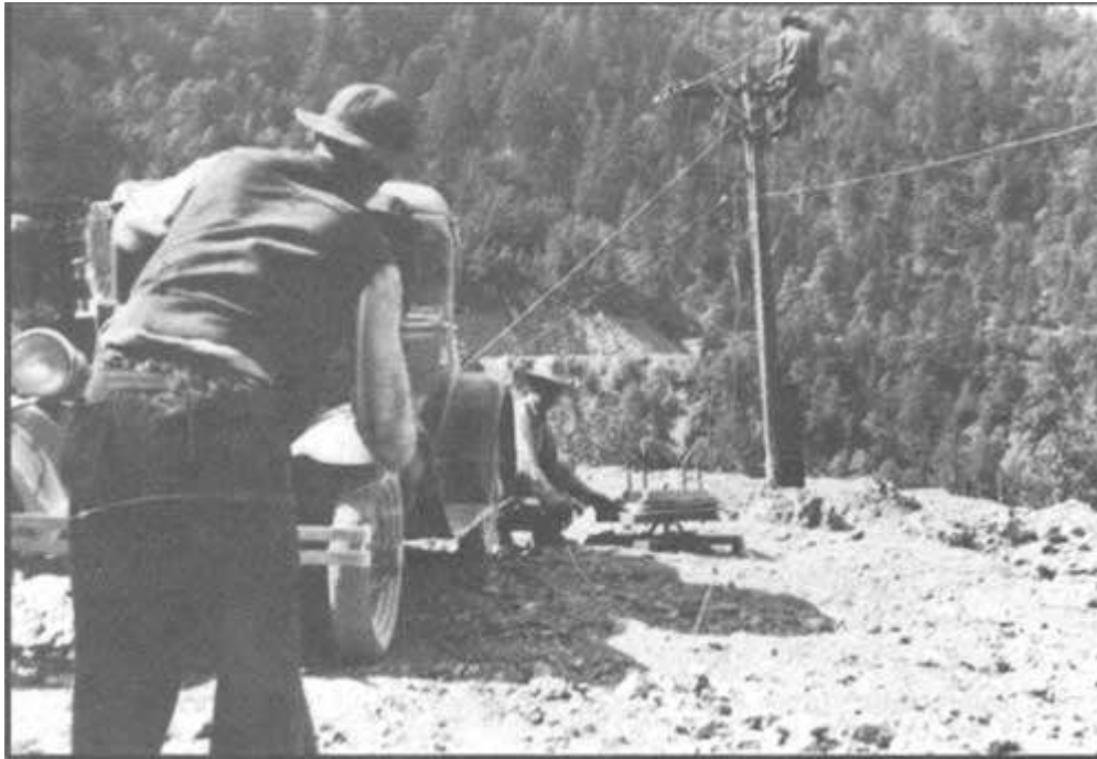
The Forest Service was often the first to bring telephone connections to remote areas. This 1934 photo shows telephone line being strung between Orleans and Somes Bar. Fred Wilder is on the reel and Lee Morford is attaching the line to the pole; the third man is unidentified. US Forest Service photo
