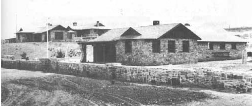
Bly District ranger station and residences built by C.C.C.
