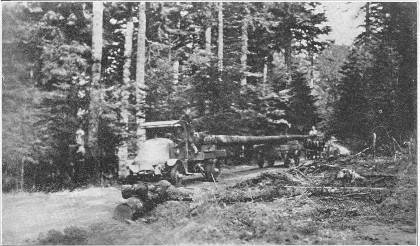
HAULING PILING 60 TO 80 FEET LONG BY MEANS OF MACK TRUCK AND TRAILER FROM THE FOREST TO THE SHIPPING POINT IN EASTERN FRANCE
