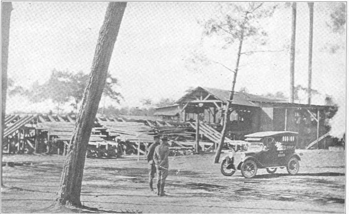
AMERICAN 20-M SAWMILL, NEAR PONTENX, LANDES, COL. BENEDICT WITH HIS BACK TURNED, IN THE FOREGROUND, STANDING NEAR NARROW GAUGE TRACK OVER WHICH LUMBER IS TRANSPORTED THREE MILES TO THE SHIPPING YARD
