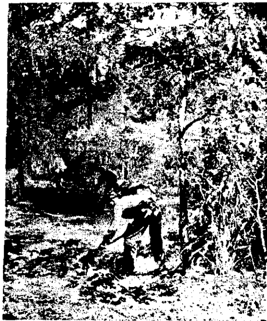
Building Fire Line
