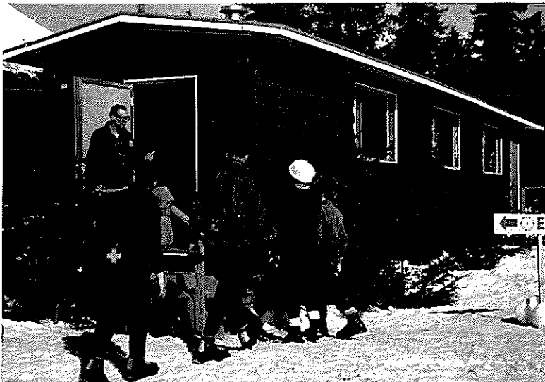
The first appearance of the Chugach Visitor Center was at Alyeska for the Olympics downhill skiing tryouts.
