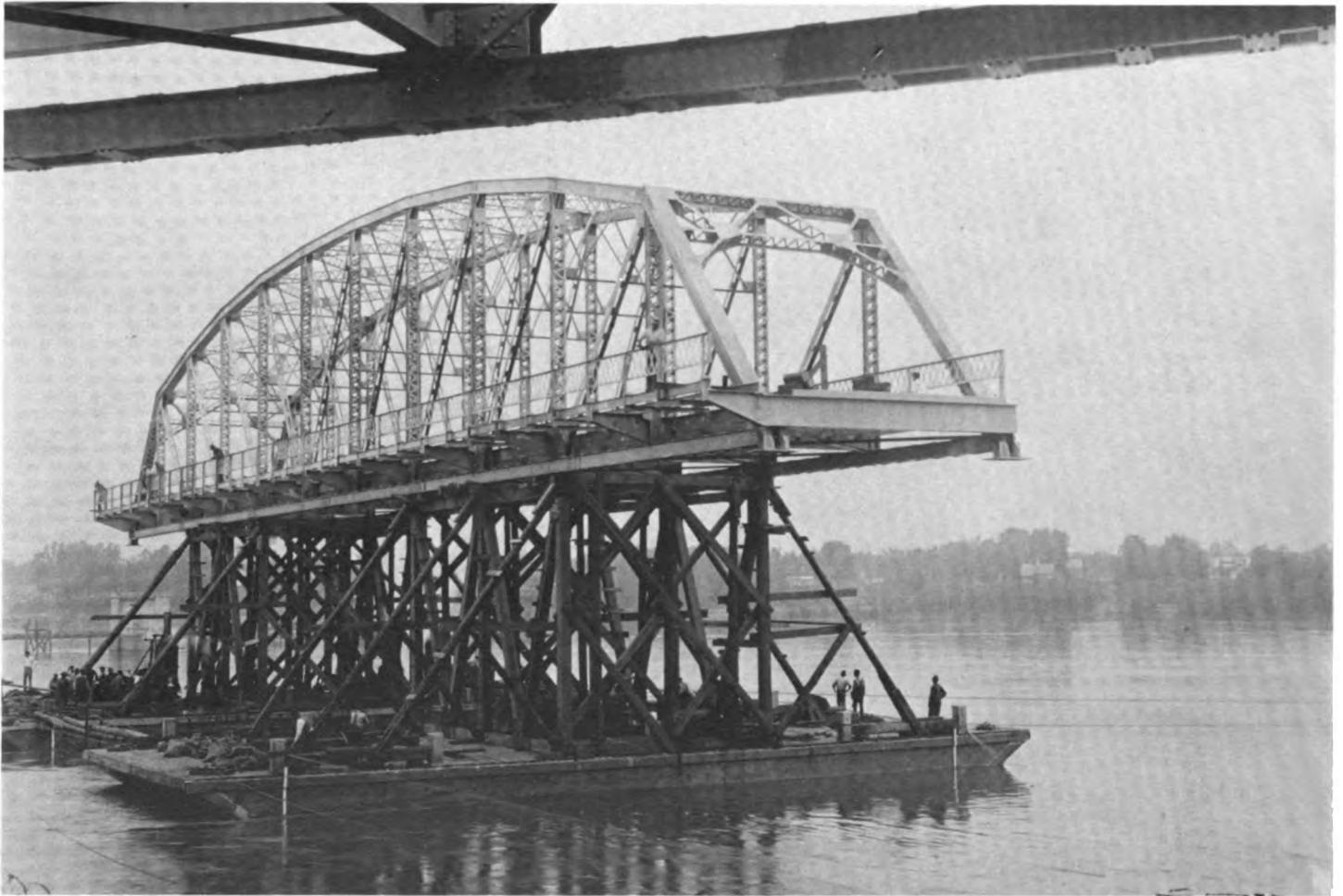
Dardanelle Bridge. The first span after being raised is turned in midstream. Once in place between piers, (photo page 73) the span is lowered to proper position. Both photographs by J.M. Wait, ca. 1928. Page 72: Photo No. 230799. Page 73: Photo No. 230800.
