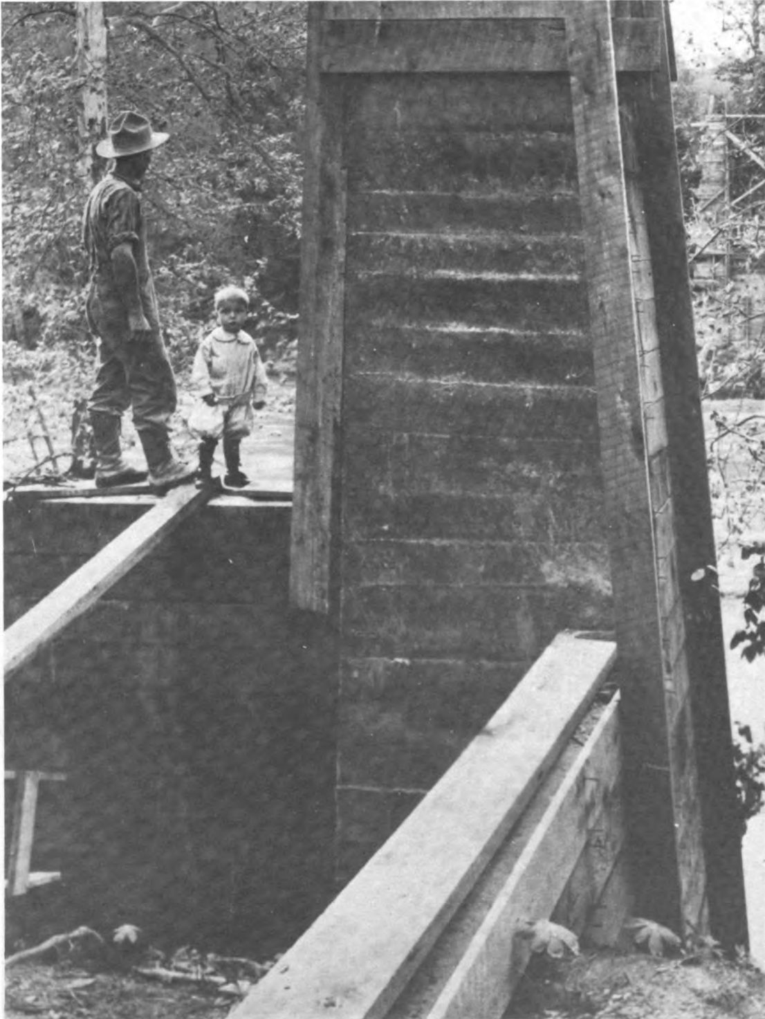
Part of south tower of Sylamore bridge. Mechanic F.A. Huey on wall. Photo No. 19509A, by Ralph Huey, 1914.
