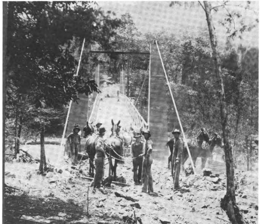
Placing cables on Sylamore bridge-concrete materials in foreground for south anchors. Photo No. 19512A, by Ralph Huey, 1914. Below: Workman on the Sylamore bridge. From an unnumbered photograph in the history files of the Ozark National Forest. Bottom photo: Sylamore Bridge. Constructed by the Forest Service and settlers. Photo No. 19756A, by Ralph Huey, 1914.
