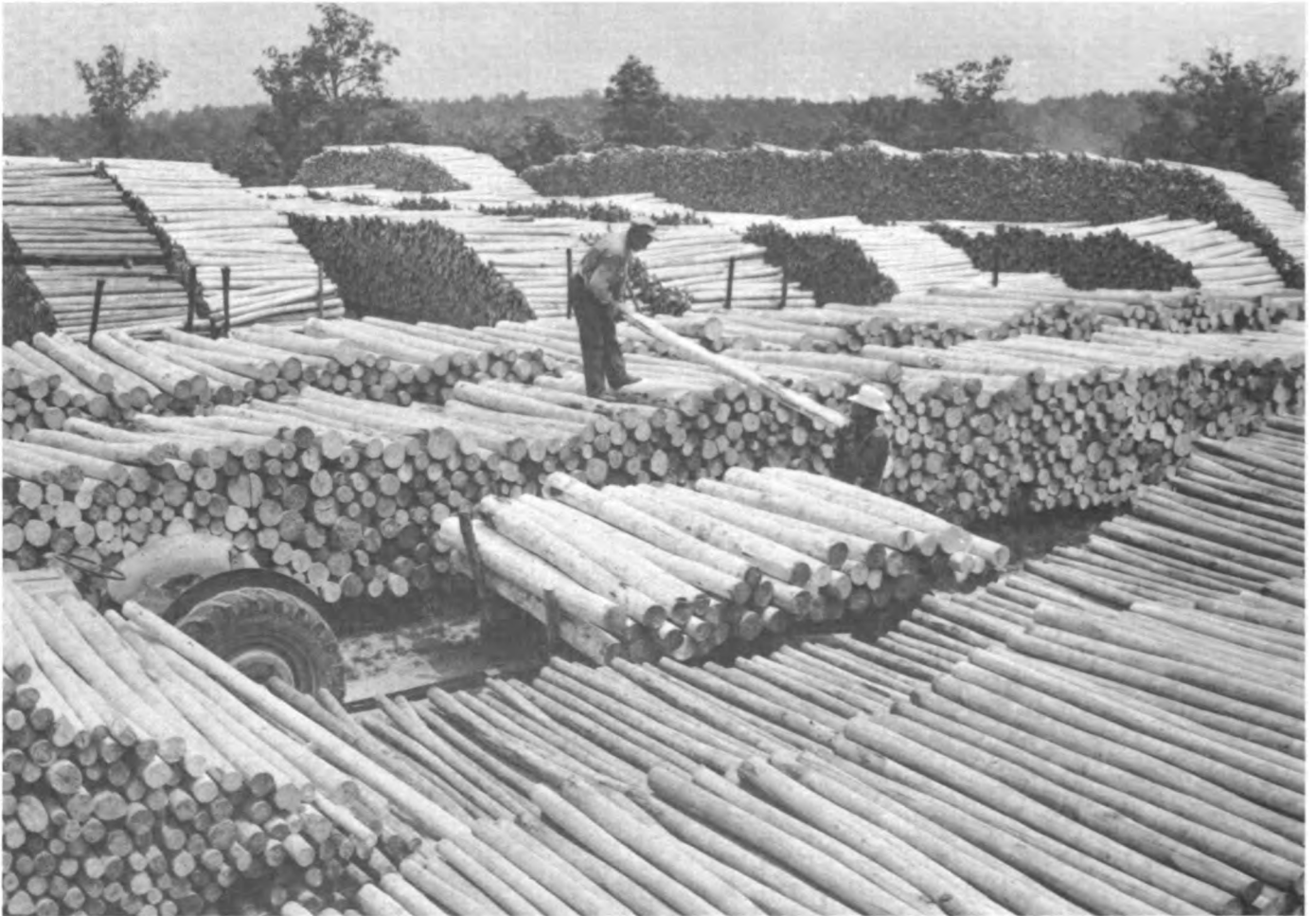
Pine post yard of the H.C. Ormond Supply Company, near Clinton, Arkansas: Much of the raw material for these posts comes from pine thinnings in the Ozark National Forest. Photo No. 505690, Daniel O. Todd, 1963.
