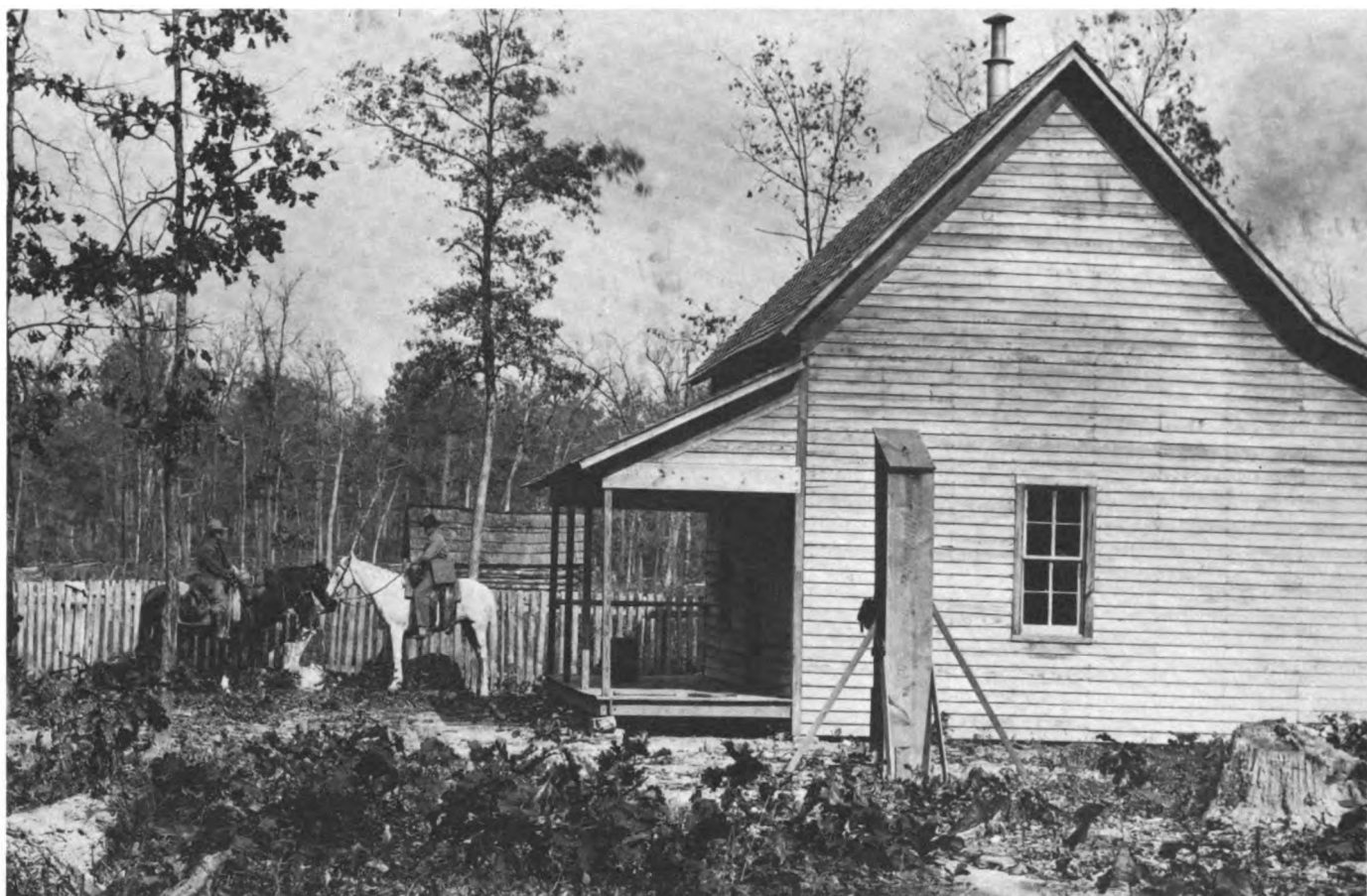
Showing proposed Rex Ranger Station. Supervisor Fitton and Ranger Vaughan mounted. Photo No. 74509, possibly by Fitton, 1908.
