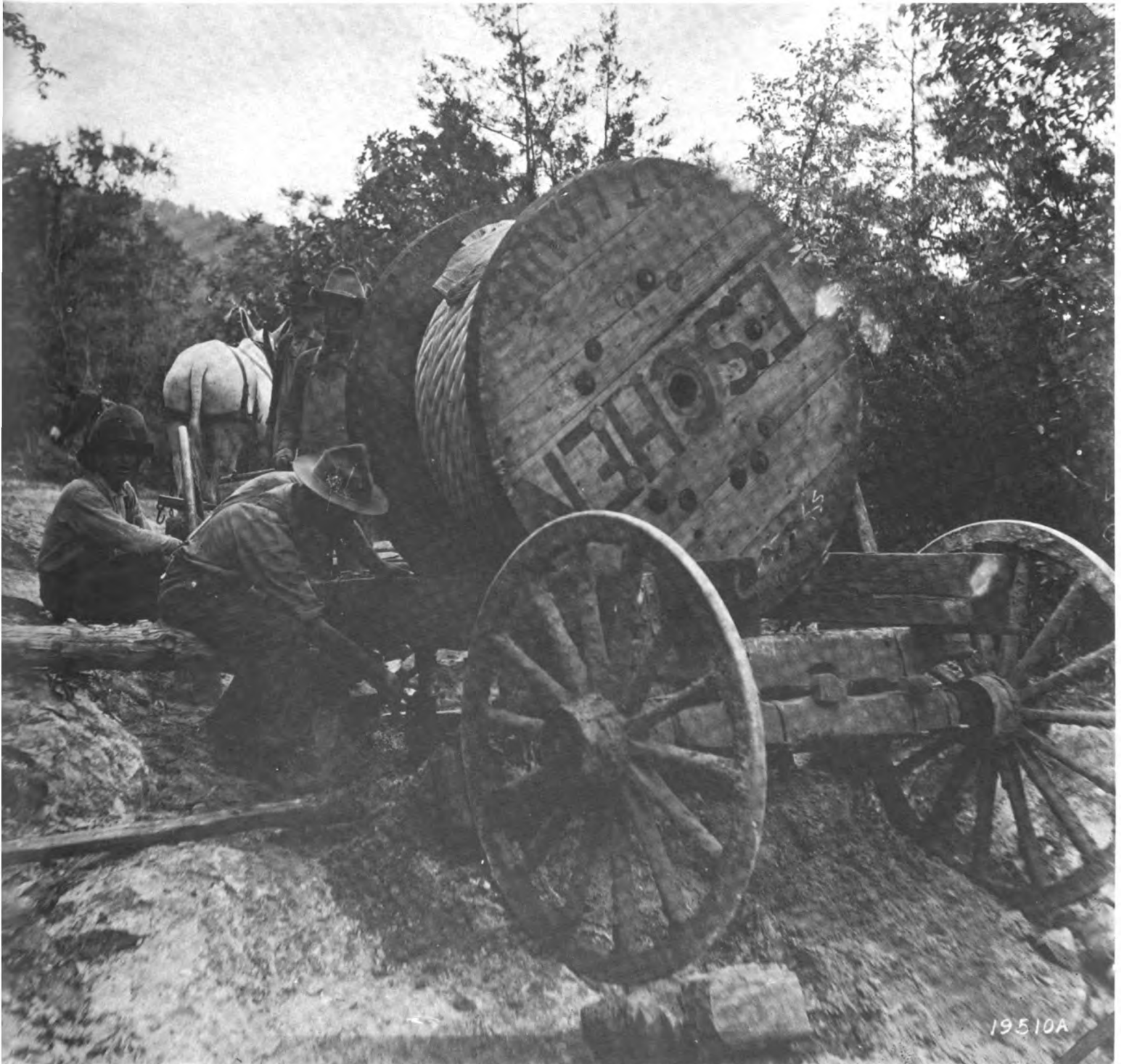
Getting over sandstone ledge with bridge cable, 4100 lbs. at stake 78, Big Flat-Sylamore Road. Front bloster and reach broken letting front end (oak railroad ties) to ground. Raising with Jack screws to put wheels under again. Photo No. 19510A, by Ralph Huey, 1914.
