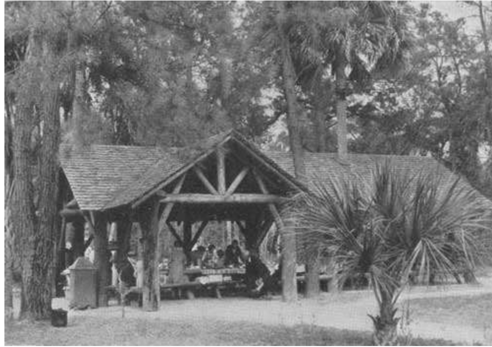
PICNIC SHELTER AT JUNIPER SPRINGS F—370107
