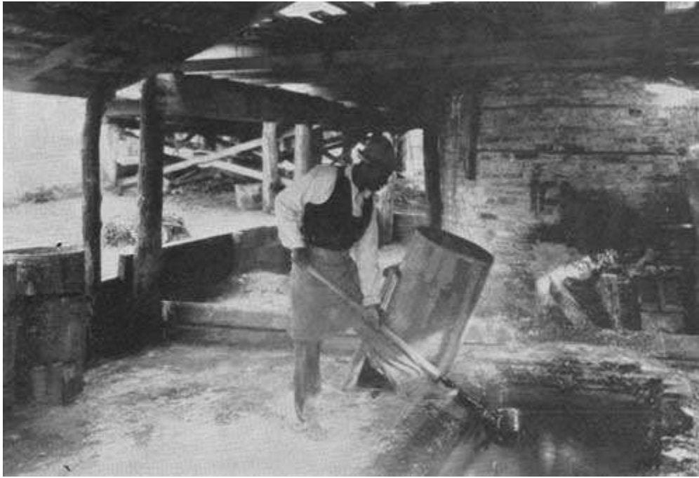
DIPPING RESIN INTO BARRELS FOR COOLING AND SHIPMENT TO THE RESIN YARD F—226771
