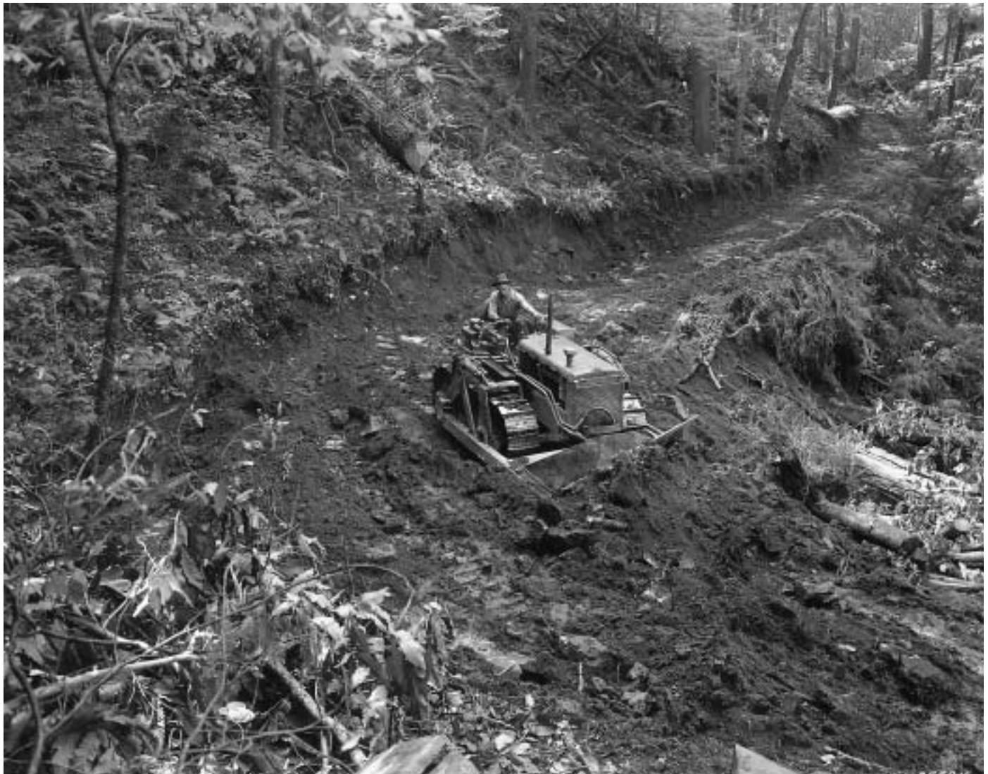
Roads on national forests increased by more than 100,000 miles from 1946–1969 as the post-World War II housing boom spurred demand for wood products. Caterpillar Diesel D4 Tractor with LaPlant-Choate trailbuilder, 1940.
