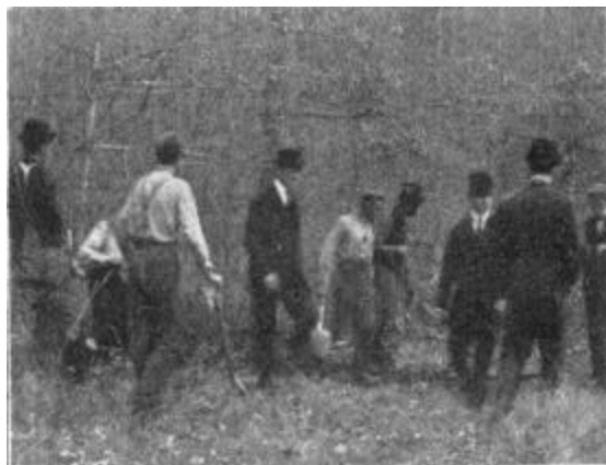
REPAIRING A BROKEN BRIDGE, AFTER PASSAGE OF PART OF THE CAVALCADE ON THE FIRST DAY OF THE FAIR.
