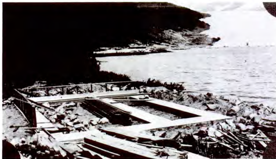
The Civilian Conservation Corps put young men to work on the national forests during the Depression. Recreational facilities built at Mendenhall Glacier near Juneau included a skaters' shelter cabin (foundation being laid in this 1936 photo) and a rifle range in the center background.
