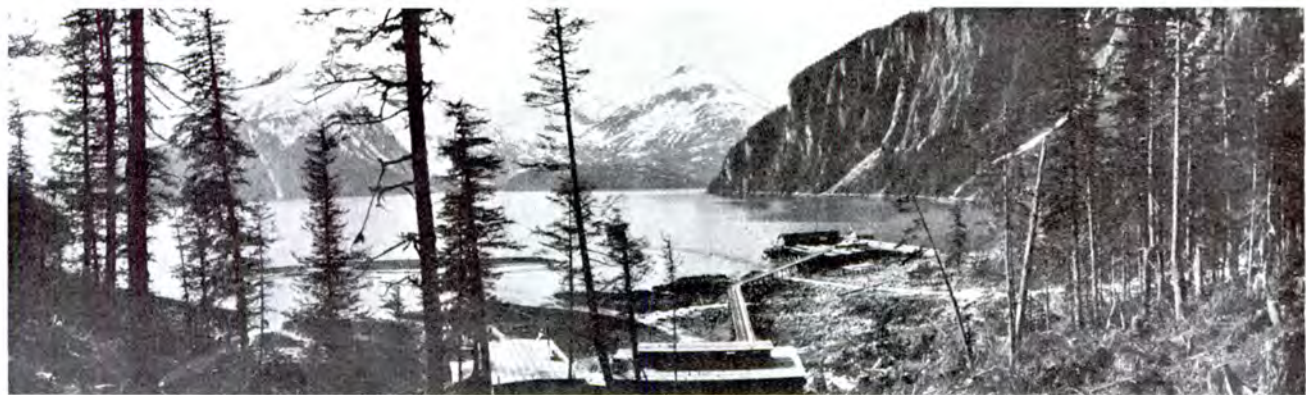
The pulp plant at Port Snettisham was doomed to failure in the early 1920s by high shipping charges and poor financial conditions.
