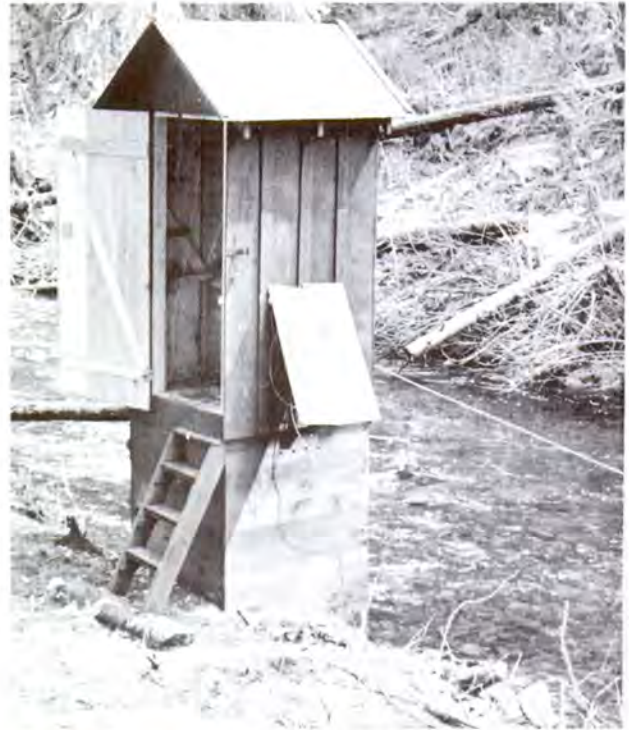
(above) The Forest Service has studied the effects of logging on salmon streams for many decades. This stream gauge on the Old Tom Creek Natural Area (part of the Society of American Foresters' system), here photographed in 1950, has been in operation since about 1940.
