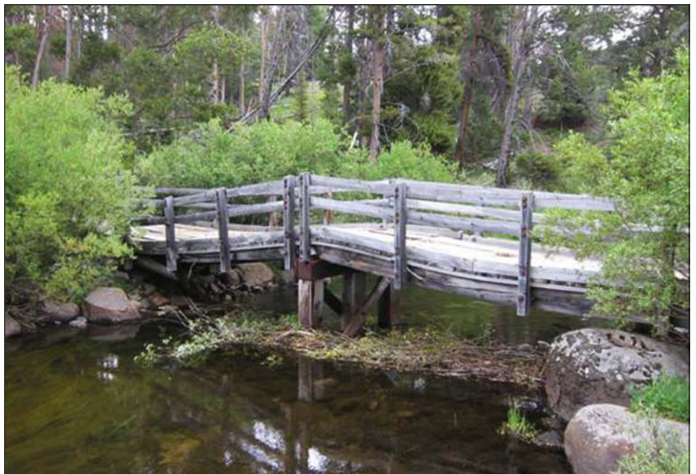
Figure 4: Example of a Failing Bridge, Beaverhead-Deerlodge National Forest, Montana
