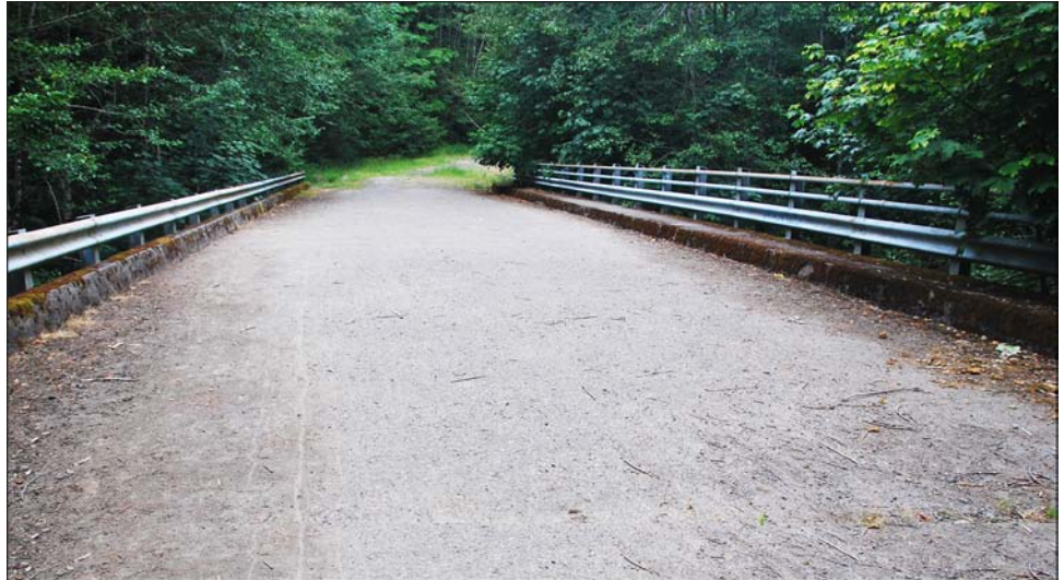
Figure 10: Road Bridge Adopted into Mt. Hood National Forest’s Trail System, Oregon
