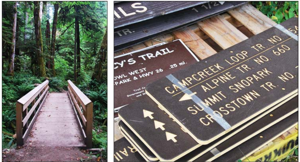
Figure 8: Bridge Replacement and Signs Paid for with Recovery Act Funding, Mt. Hood National Forest, Oregon
