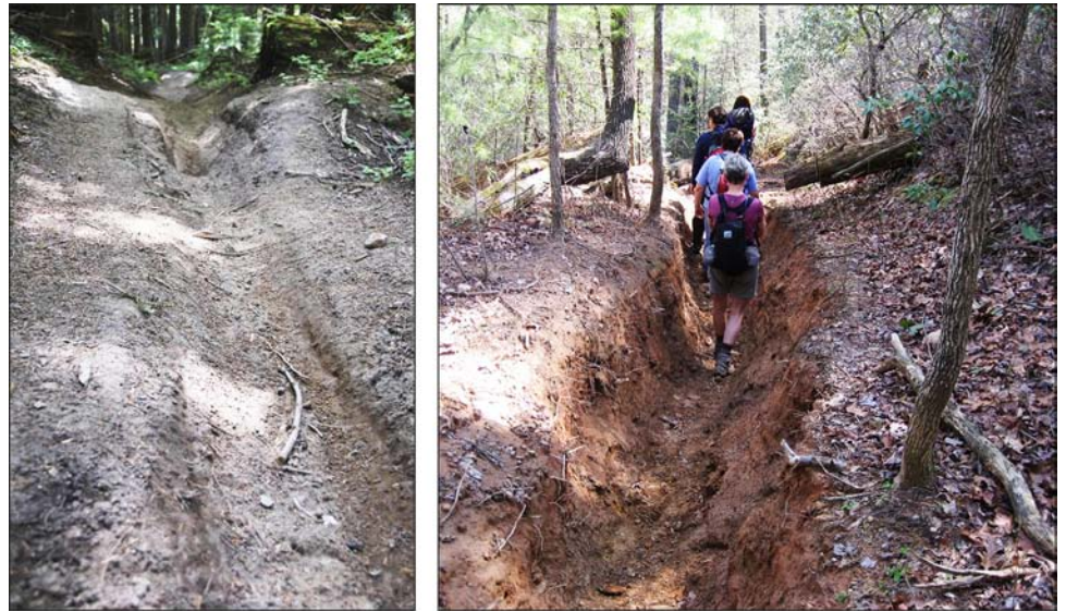
Figure 6: Deep Trenches Due to Inadequate Drainage, Gifford Pinchot National Forest, Washington, and Chattahoochee-Oconee National Forest, Georgia
