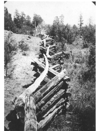
Figure 4. Hand-split rails stacked in zigzag fashion were commonplace across early America. Fences such as the one above, consumed large quantities of wood and deteriorated quickly. Forest History Society photo.
