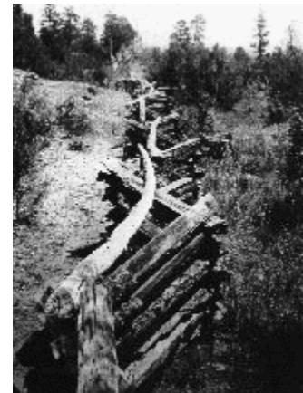
Figure 4: Worm Fence A quick way to fence livestock was the worm fence. In order to avoid digging postholes, timbers were stacked atop each other in a zigzag pattern. These were poorly made, required a huge quantity of wood, were subject to rot, and had to be replaced every 6 to 8 years. Forest History Society photo.
