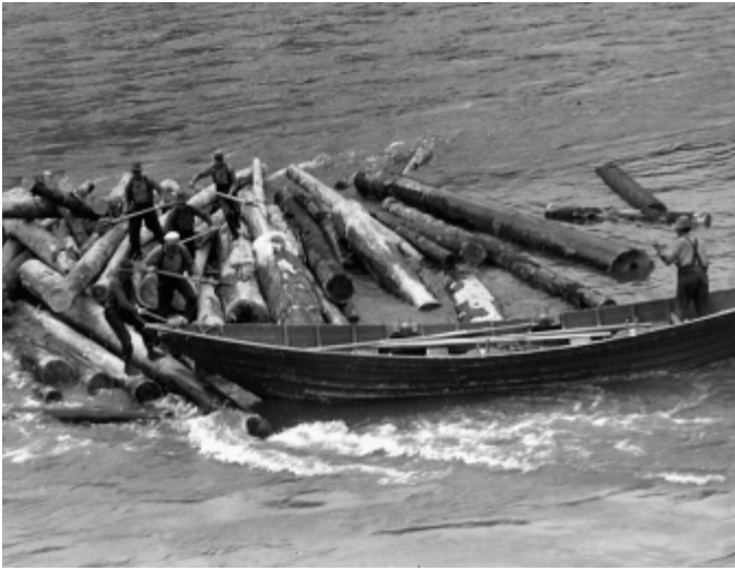
“Head’s Up, she’s a pullin’.” The bateaux crew pulling a small center jam in the North Fork of the Clearwater River. The men in the picture are leaping to the safety of the bateaux as everything is moving and the jam is breaking up.
