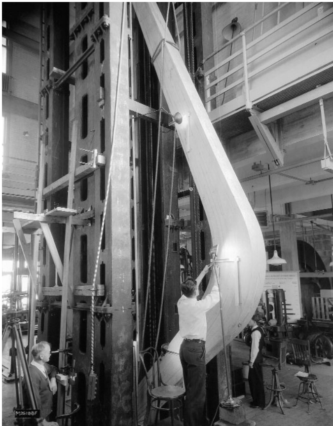
Research at the Forest Products Laboratory brought the use of glued-laminated timber to the United States in the 1930s. This photograph was taken for Mr. T.R.C. Wilson on January 14, 1935. Wilson was an early FPL researcher who did extensive work on wood arches and other structural components. This is glulam arch D-1 in a testing machine.
