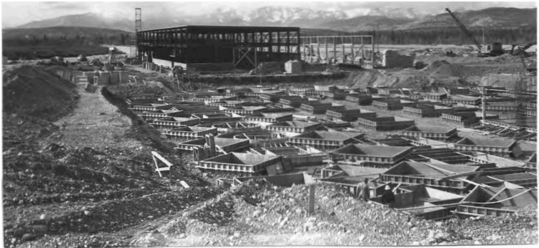
The Hinton, Alberta mill under construction. Photo courtesy St. Regis Paper Company.
