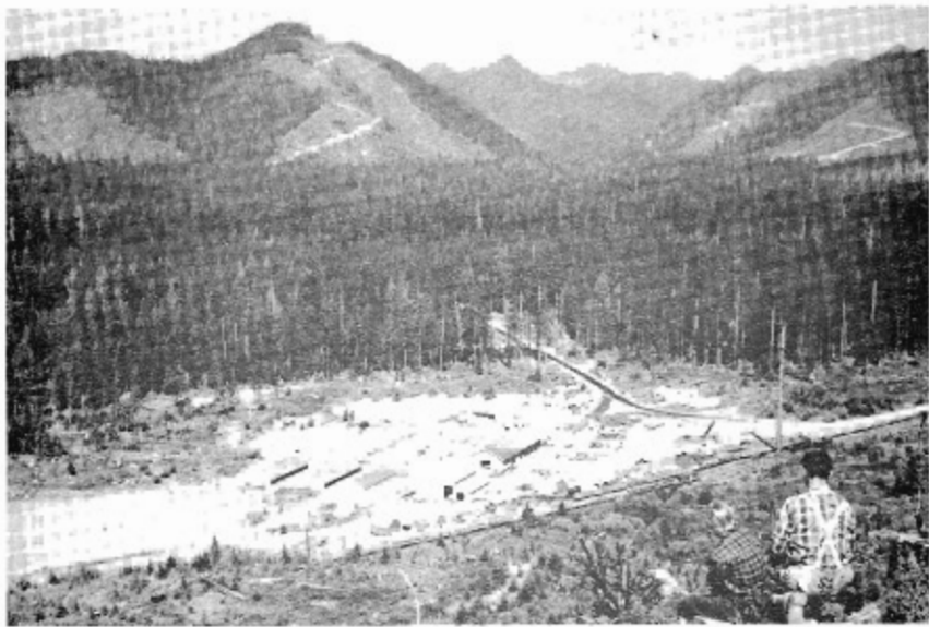
Simpson's Camp Grisdale, forty-seven miles west of Shelton, Washington. It is one of the large remaining bunkhouse logging camps in the West.
