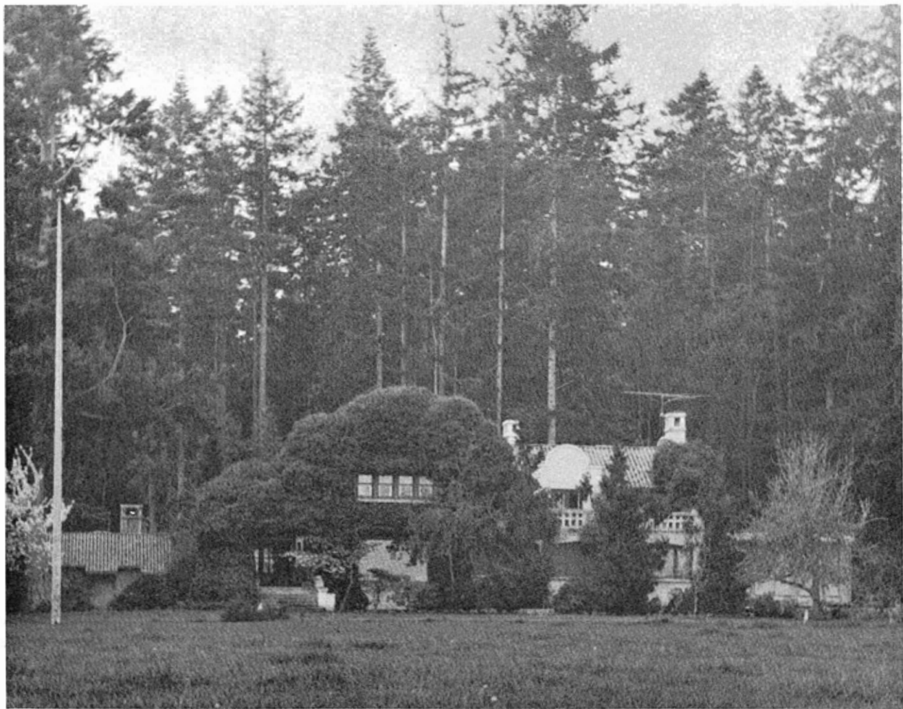
Main residence (locally called the "Anderson Mansion") at Grays-marsh before removal of ivy. February 1977.
