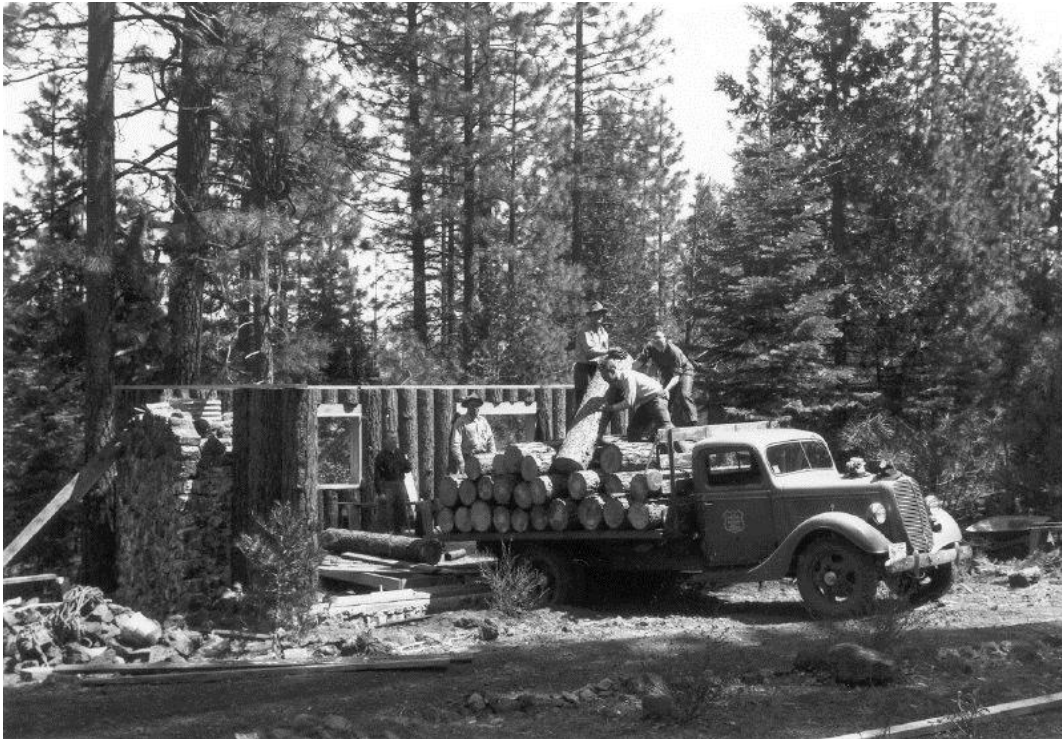
Because funds for construction were lacking, staff of the Berkeley Forest Insect Lab built a bunkhouse in 1943 at Hat Creek Field Station, Lassen County, CA, with treated logs as an "experiment." The stated purpose was to see how long bark would be retained. They are (l. to r.): R.C. Hall, "Shorty" Startt, G.R. Struble, J.W. Bongberg and P.C. Johnson.
