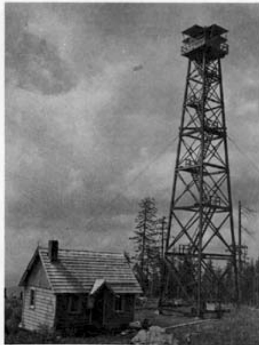
1937 photograph of fire tower in Washington state.
