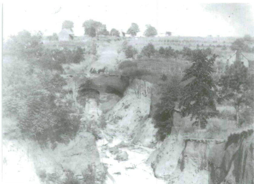
Figure 4. Gully that, this photograph suggests, was the product of road drainage. Courtesy of Sam Singer.
