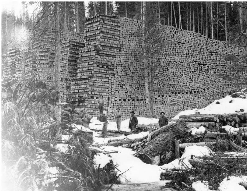
Figure 9. Railroad bridges and trestles (top) were constructed of pilings and large timbers. Railroads consumed vast quantities of wood, as these stacked cross-ties show (bottom).
