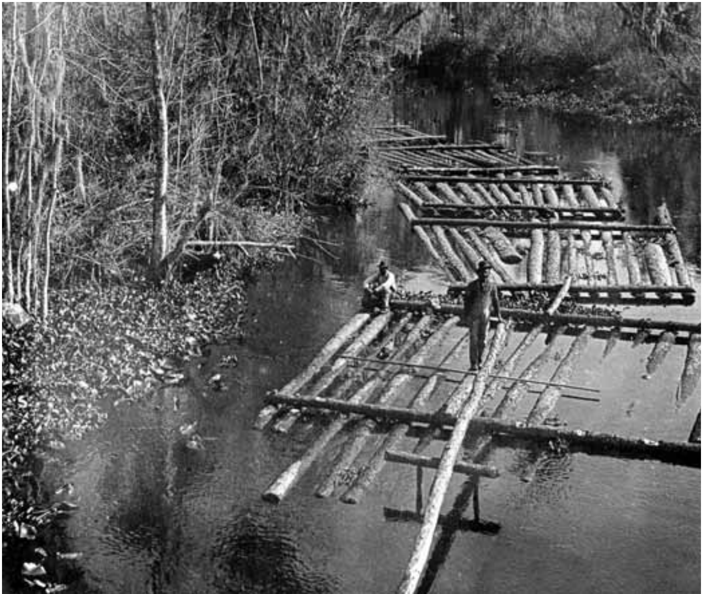
On the Oklawaha River in 1901, rivermen moved cypress logs cut in the swamps of central Florida and rafted them downriver to mills. The two front sections of the rafts pivoted to make navigating the winding river easier. The Oklawaha flows northward into the St. Johns River, both of which were used for transporting lumber to market in Jacksonville.
